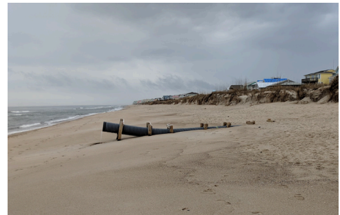
Photo 1: Davis Road Stormwater Outfall During Discharge Event
