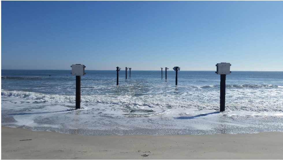
Fig. 3 Outfall buried and extended beyond the surf zone, and marked with warning signs
