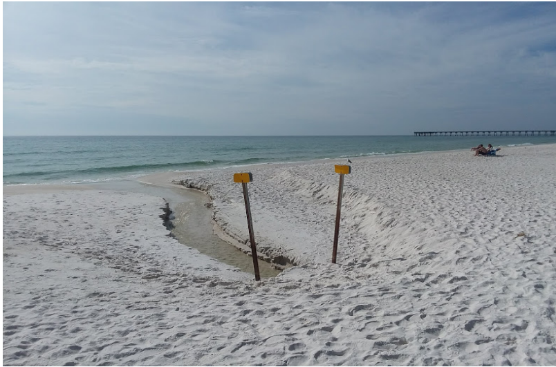
Fig. 1 Non-extended outfall on a nourished beach
