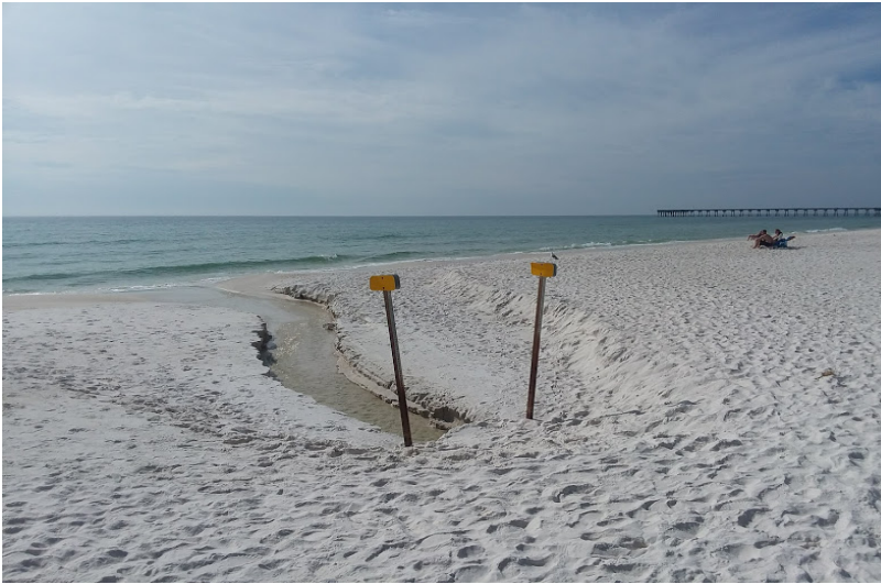
Fig. 1 Non-extended outfall on a nourished beach
