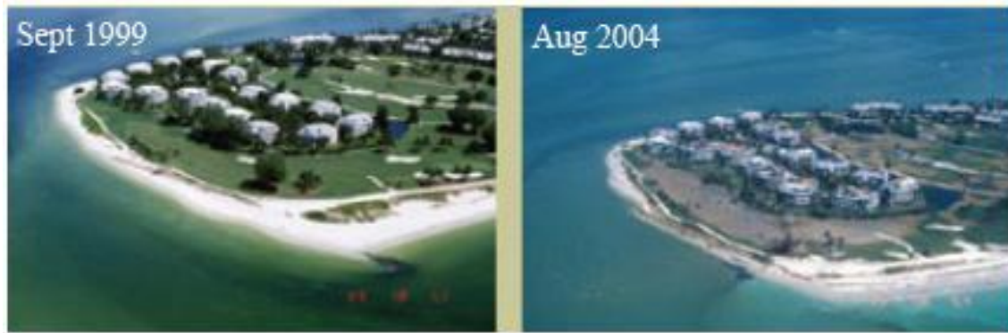
Figure II-59. Comparison of Photographs Taken Before and Immediately After the Passage of Hurricane Charley Showing Beach Erosion Inside the Inlet
