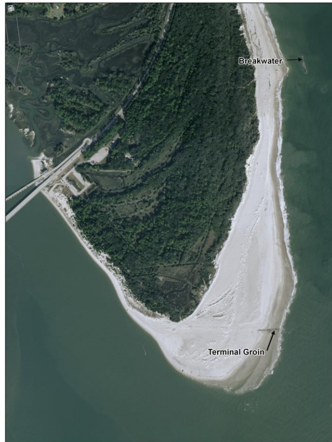
Figure II-41. Amelia Island Terminal Groin and Breakwater
