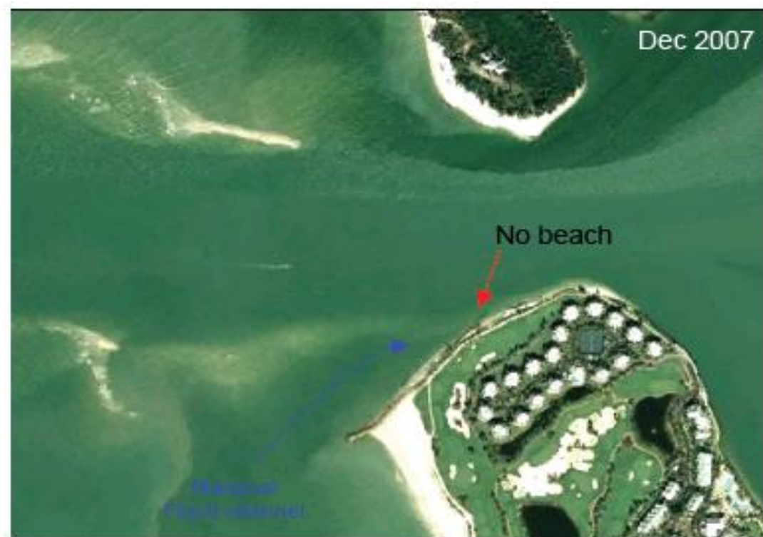
Figure II-56. View of the Terminal Groin at Redfish pass (from Google Earth)
