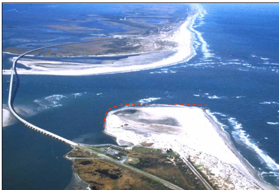
Figure II-6. Oregon Inlet Terminal Groin & Revetment
