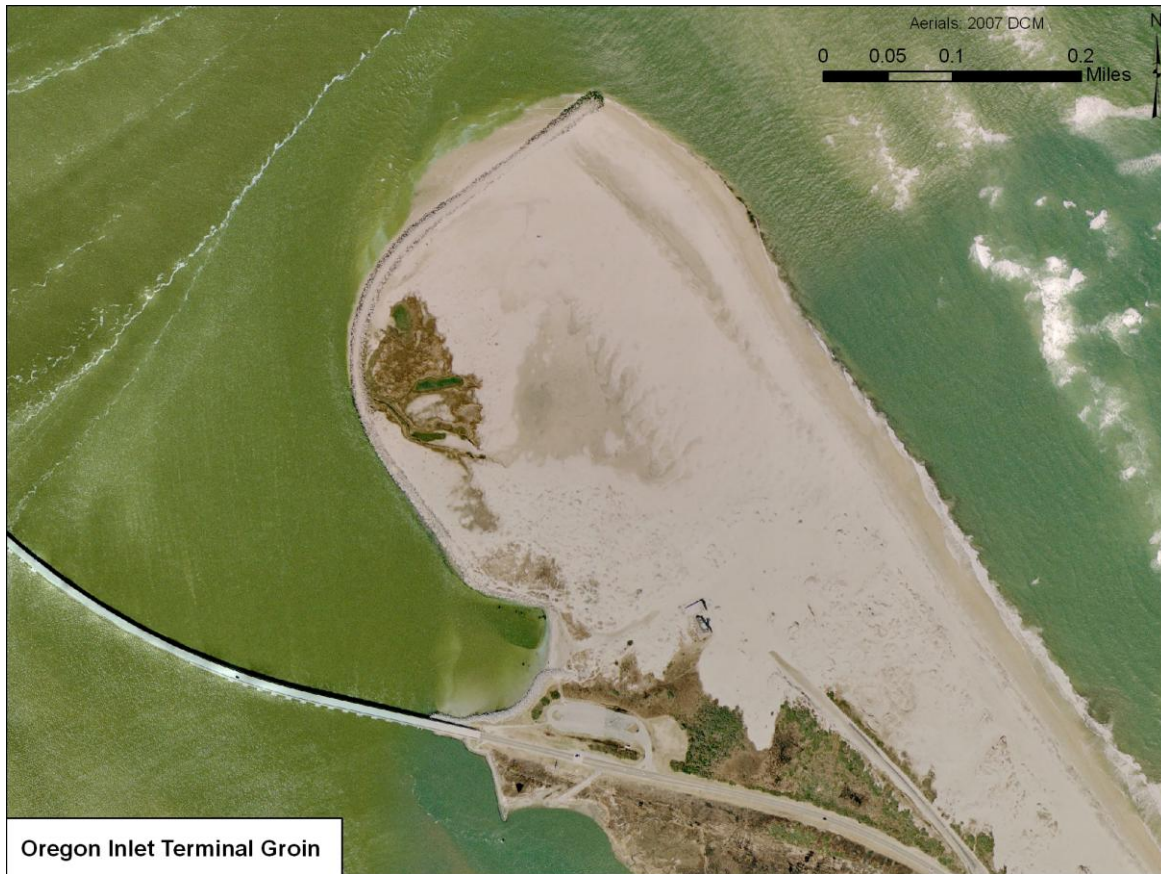
Figure III-1. Oregon Inlet Terminal Groin and Revetment
