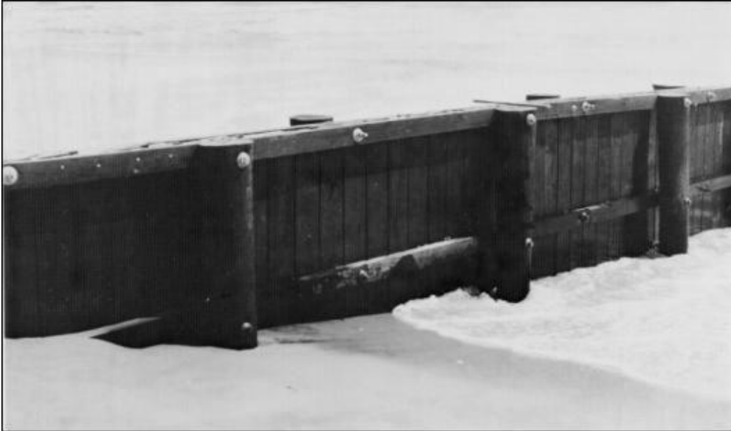
Figure VI-6. Example of a Timber Groin
