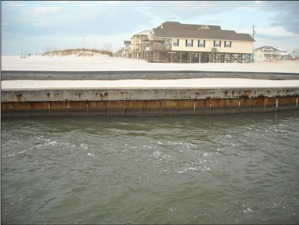
Figure VI-4. Example of Concrete Sheet Piles
