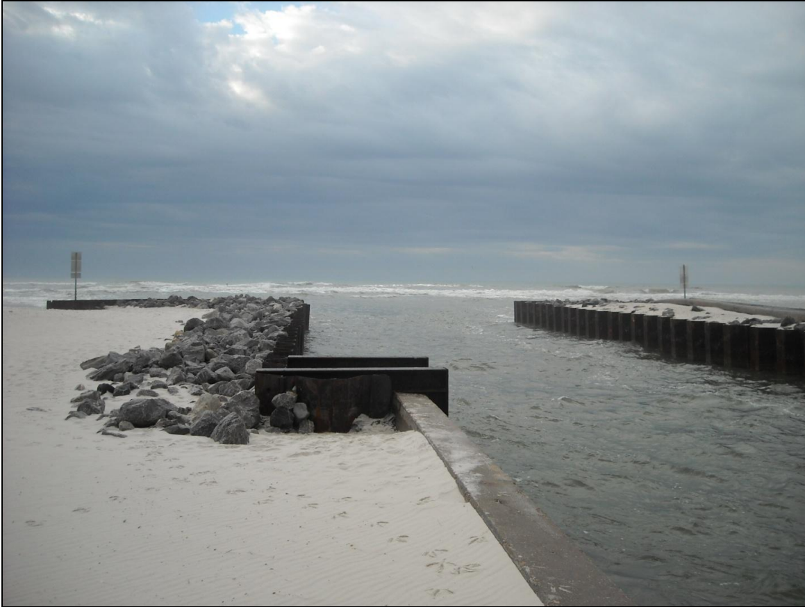
Figure VI-5. Example of Steel Sheet Pile Terminal Groins
