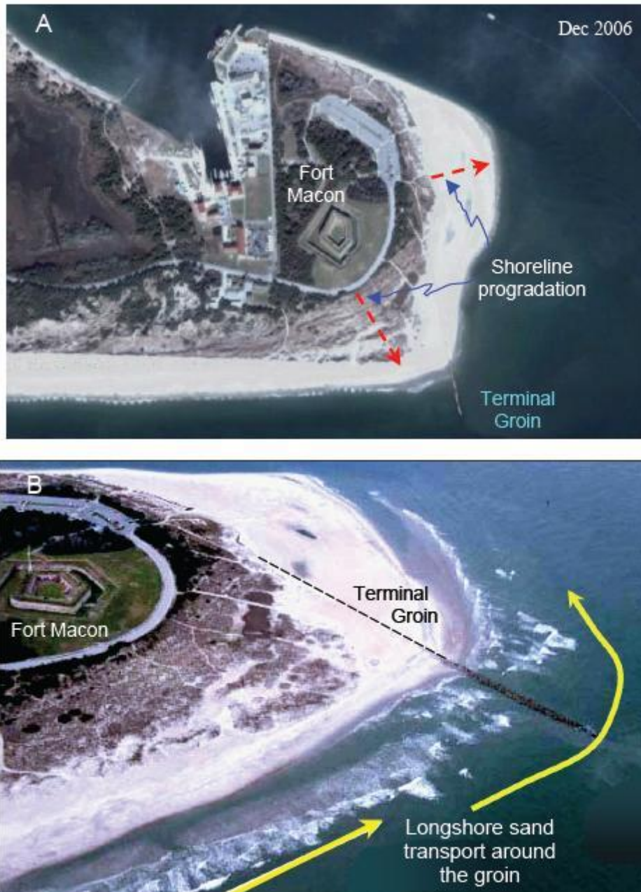
Figure III-20. Photographs Illustrating Progradation of the Beach West of the Groin and Along Inlet Shore. Dashed line indicates extent of groin beneath the beach
