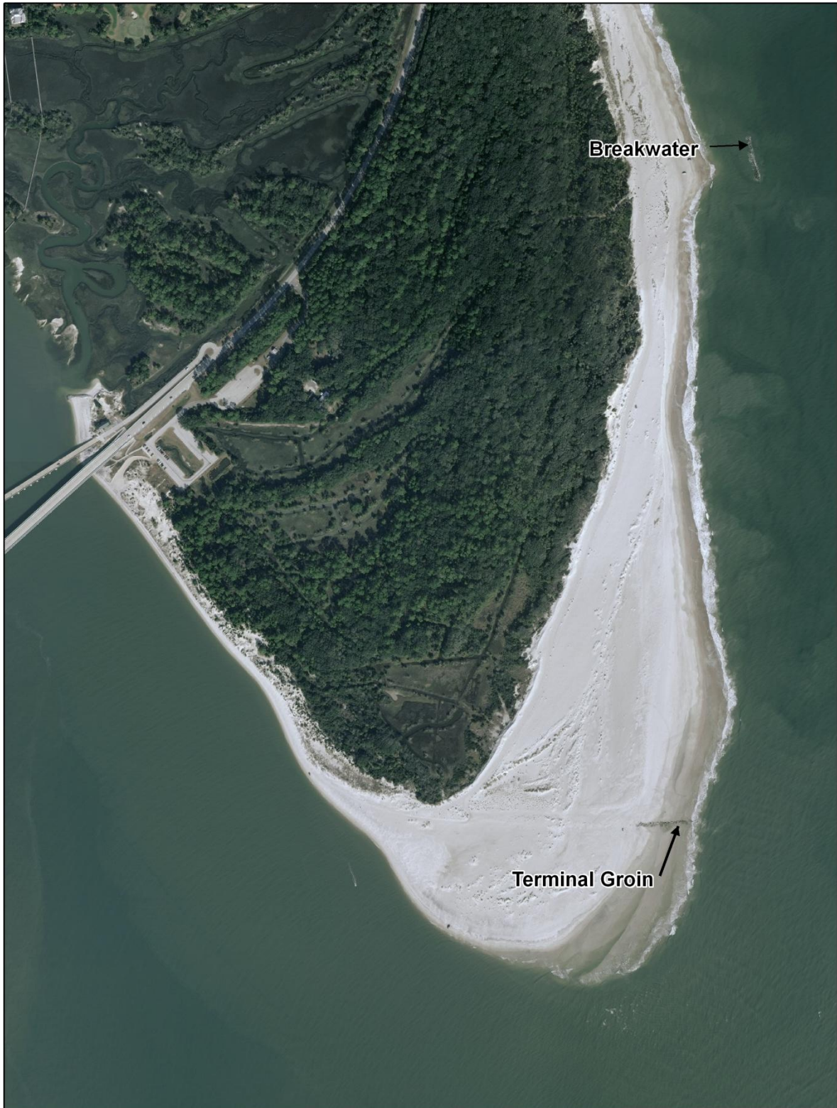
Figure V-6. Amelia Island Terminal Groin
