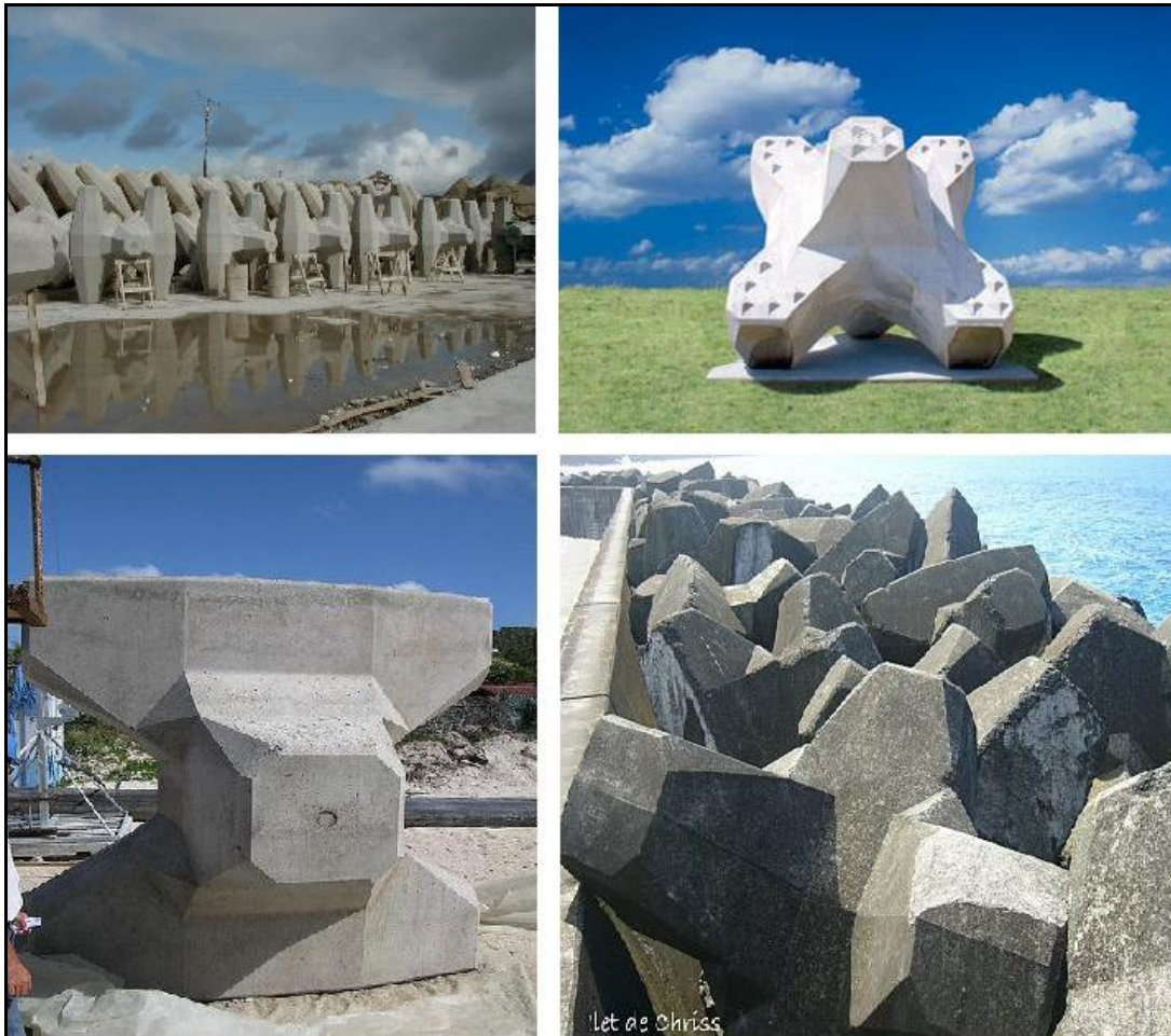
Figure V-27. Examples of Concrete Armor Units
