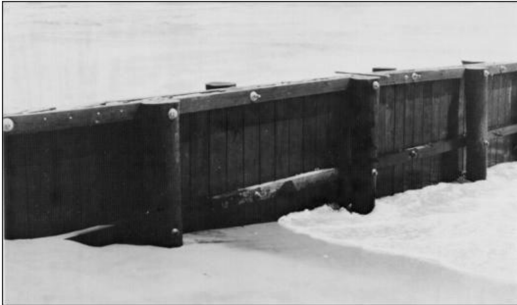
Figure V-29. Example of a Timber Groin
