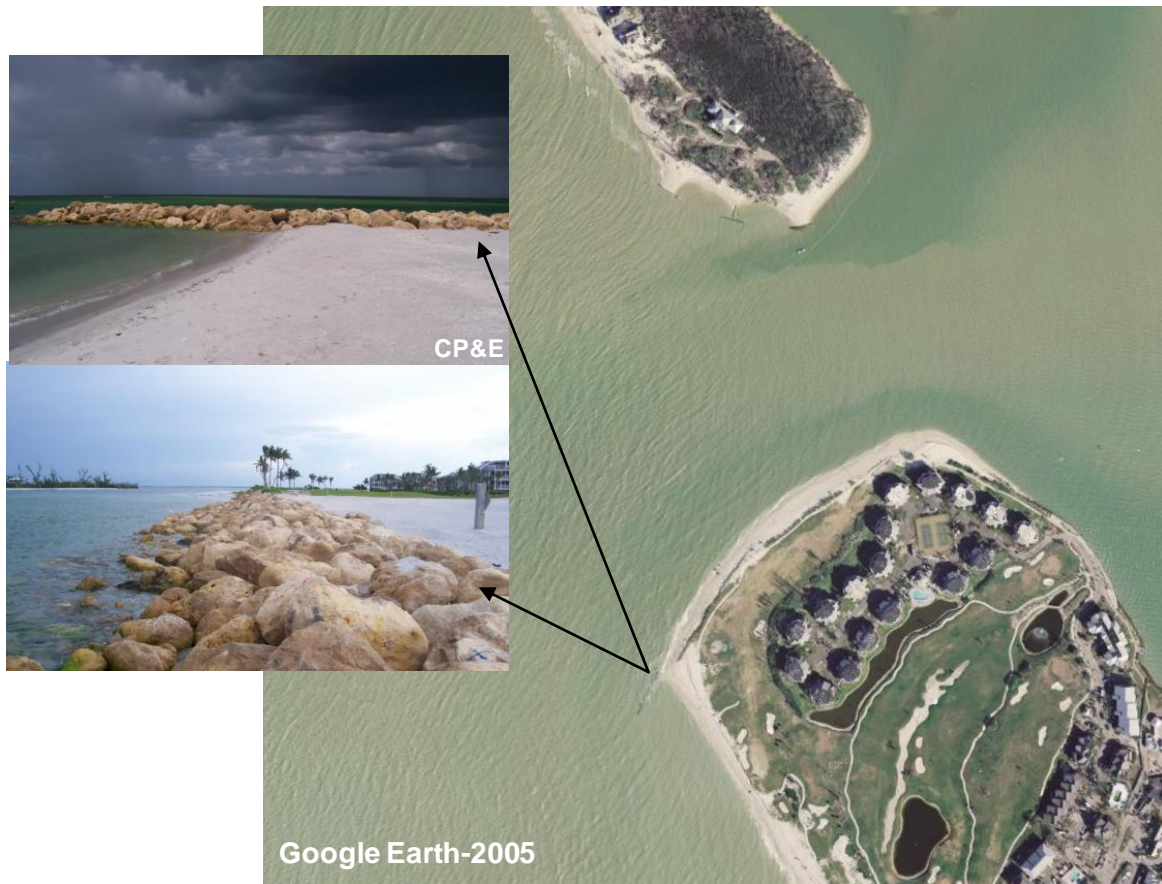
Figure II-40. Terminal Groin Rehabilitation
