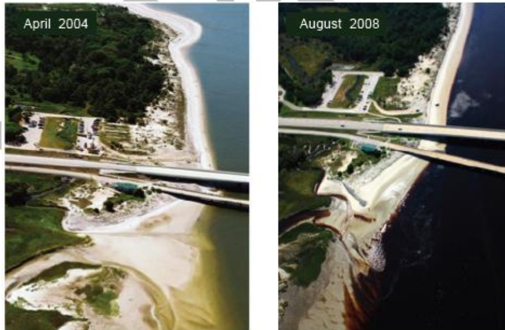
Figure III-29. Photographs Showing Before and After the Construction of the Backside Terminal Groin (Olsen, 2008)
