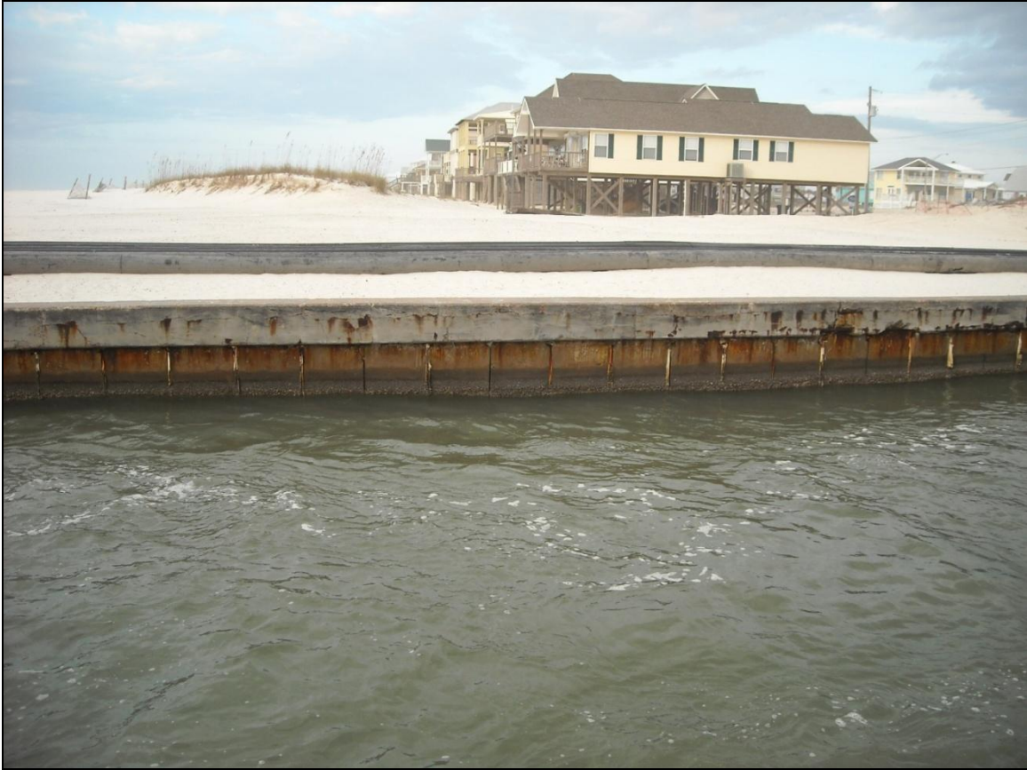
Figure V-26. Example of Concrete Sheet Piles
