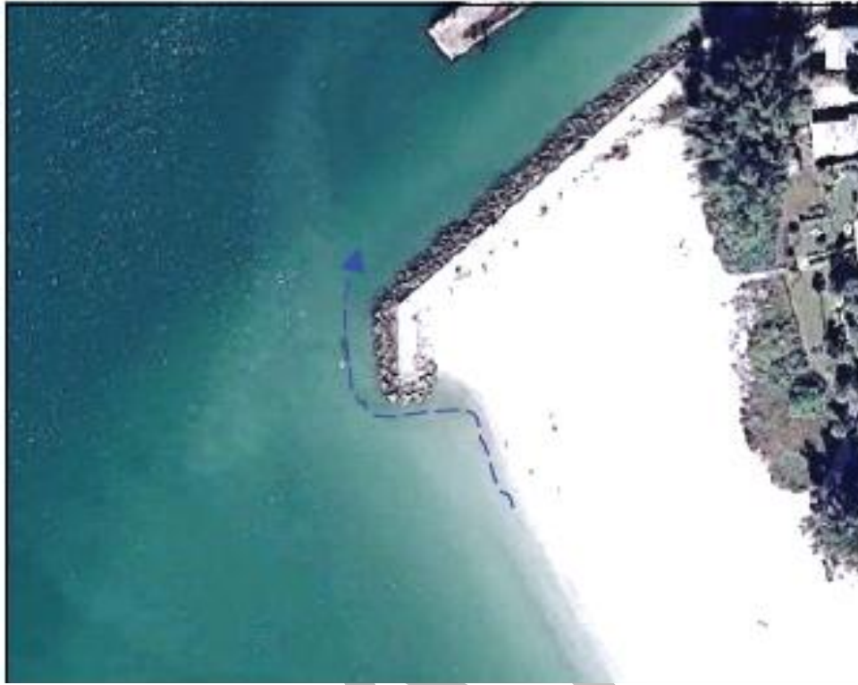
Figure III-42. Vertical Aerial Photograph of the Terminal Groin at the South Side of John's Pass at the Northern End of Treasure Island (from Google Earth)
