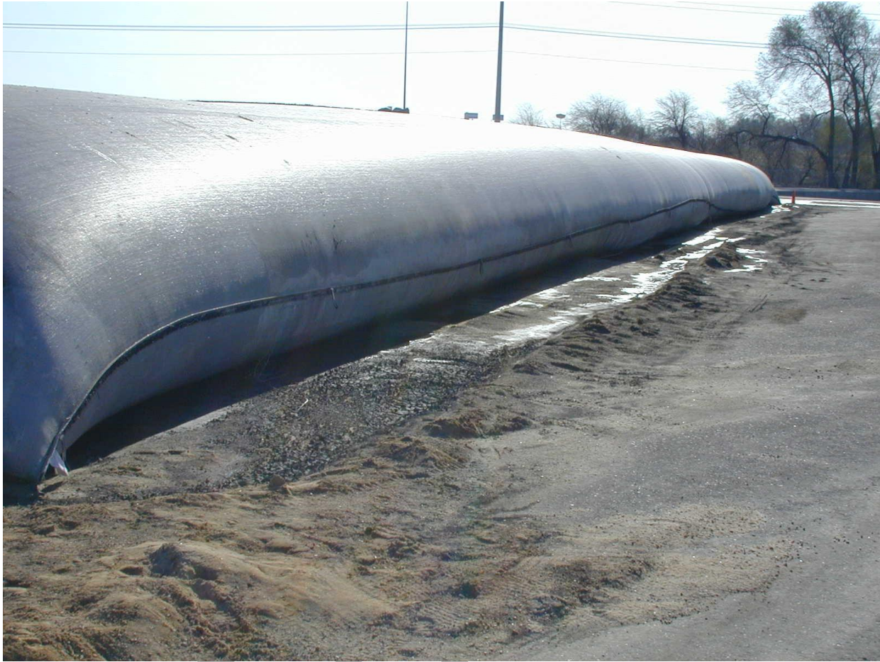
Figure V-30. Example of a Geotextile Tube
