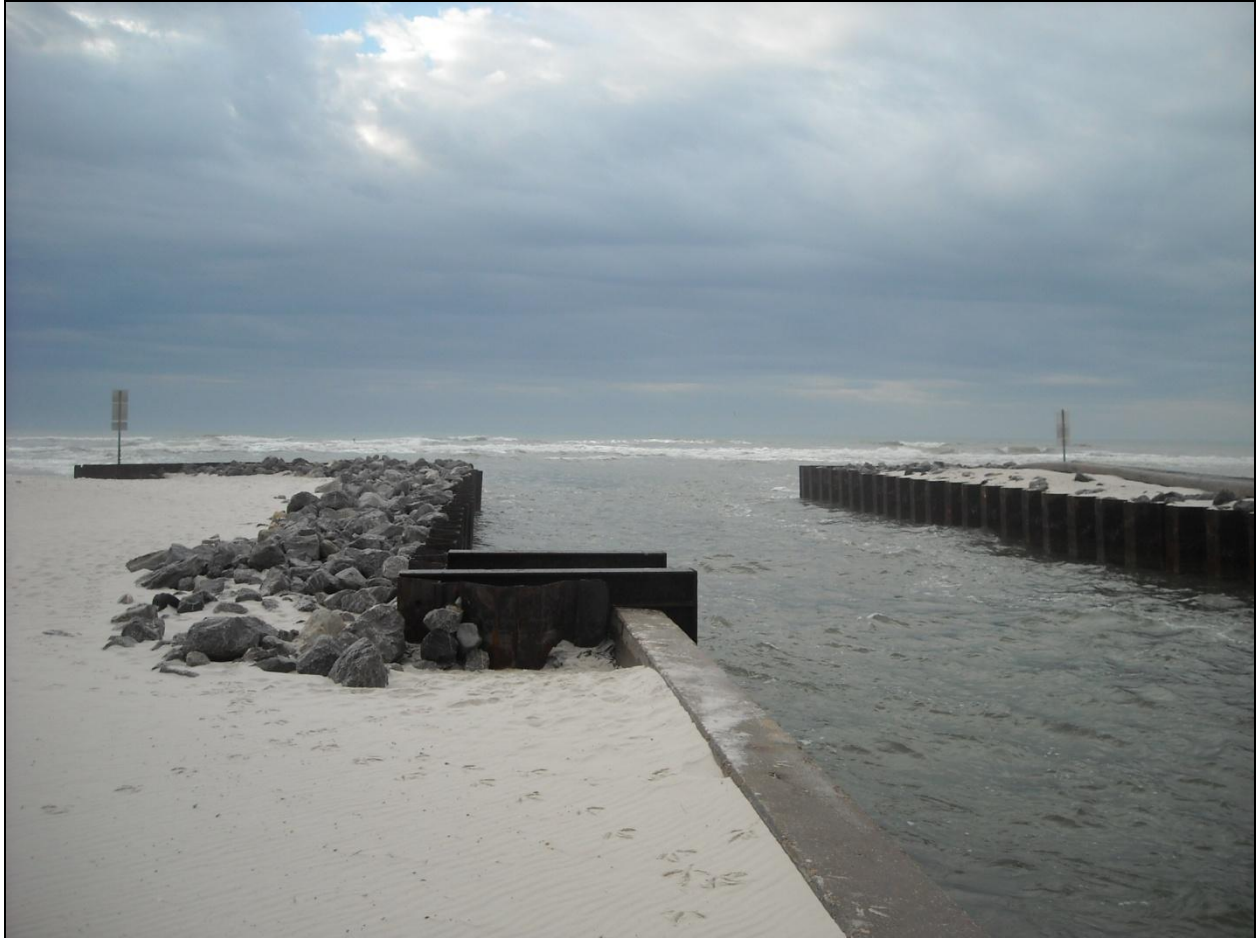
Figure VII-5. Example of Steel Sheet Pile Terminal Groins
