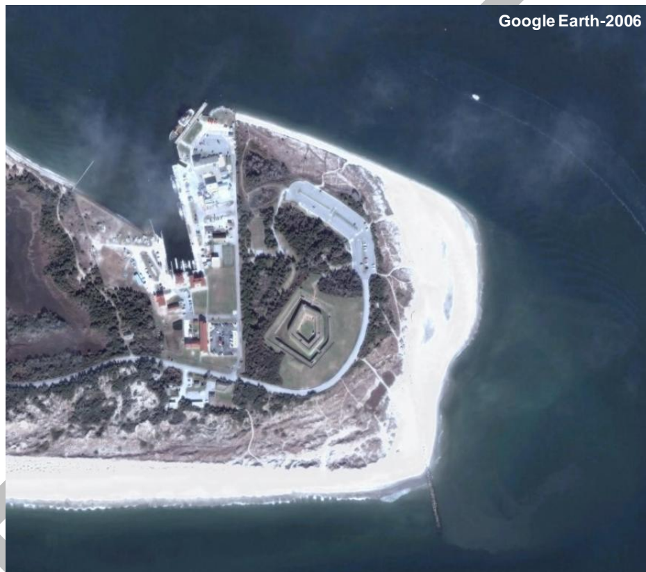
Figure II-13. Fort Macon Terminal Groin
