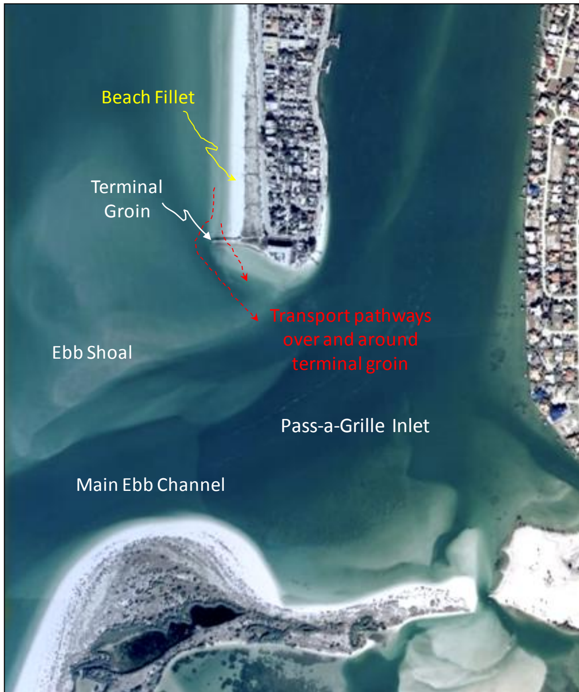
Figure III-1. Terminal Groin at Saint Pete Beach, Florida
