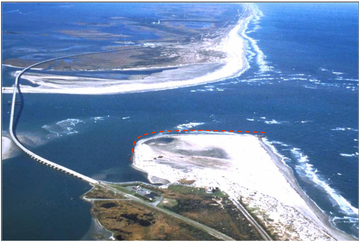
Figure II-1. Oregon Inlet Terminal Groin
