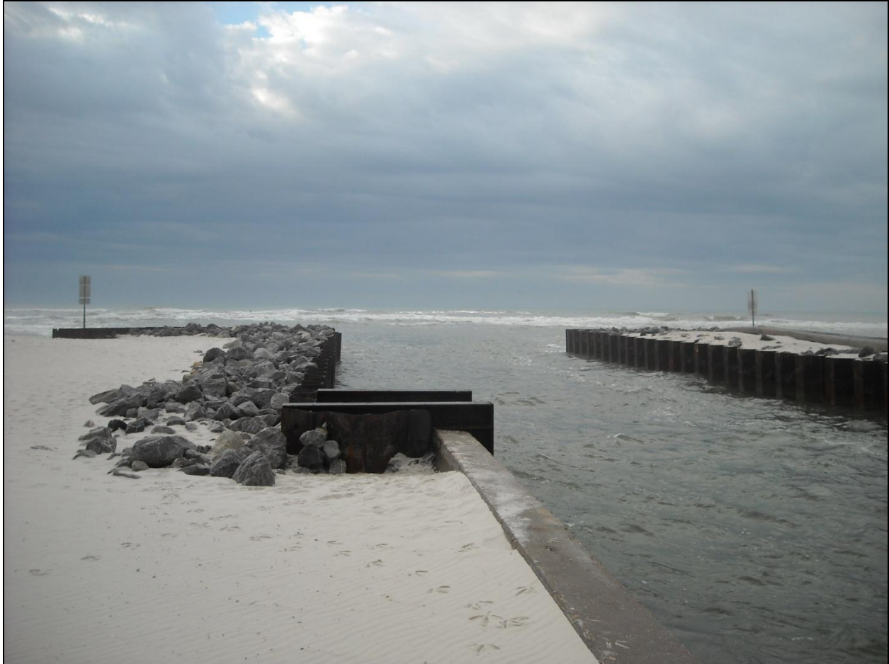
Figure V-28. Example of Steel Sheet Pile Terminal Groin
