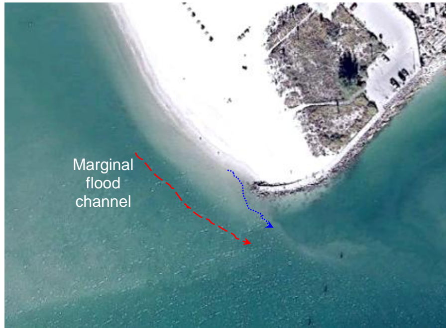
Figure III-41. Vertical Aerial Photograph of the Terminal Groin at the North Side of John's Pass
