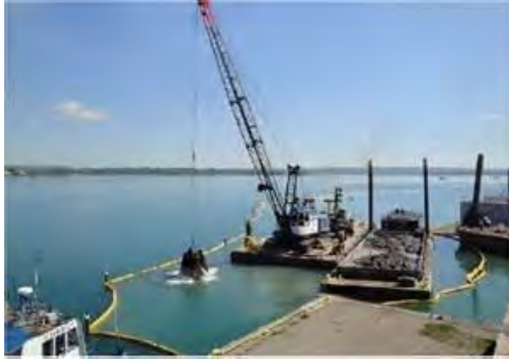
Figure 4. Photograph of Mechanical Dredging
