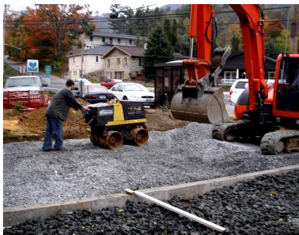
Figure 12. Aggregate Placement and Compaction (NCSU-BAE)
