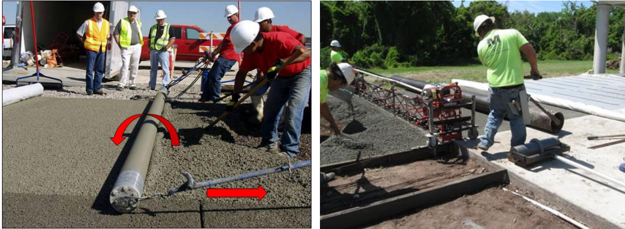
Figure 14. Compacting Pervious Concrete (NCSU-BAE)
