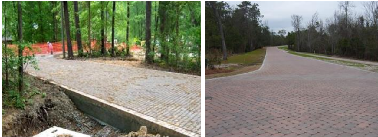
Figure 5. Edge Restraints on PICP
