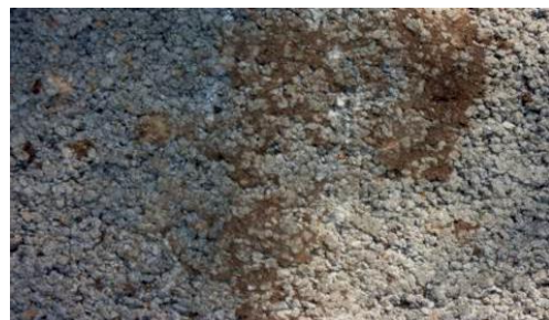
Figure 15. Clogged Pavement
