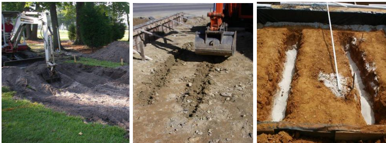
Figure 10. Good Construction Practices, from left to right: Grading from the Side (NCSU), Scarifying the Subgrade (Tyner), Trenching the Subgrade (Tyner)
