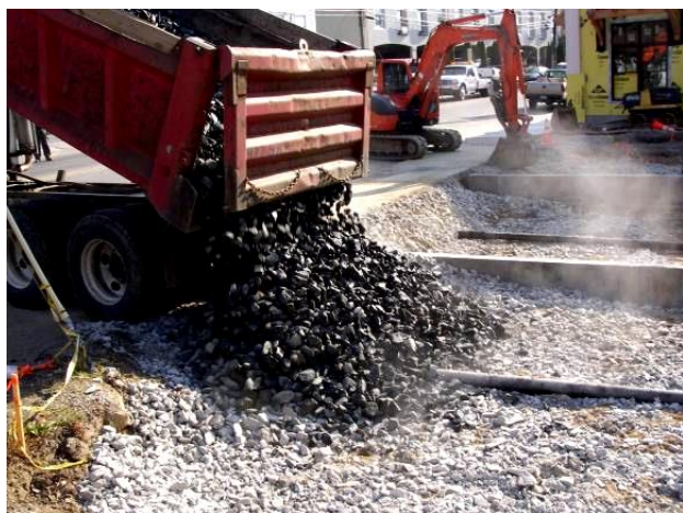
Figure 12. Aggregate Placement and Compaction (NCSU-BAE)
