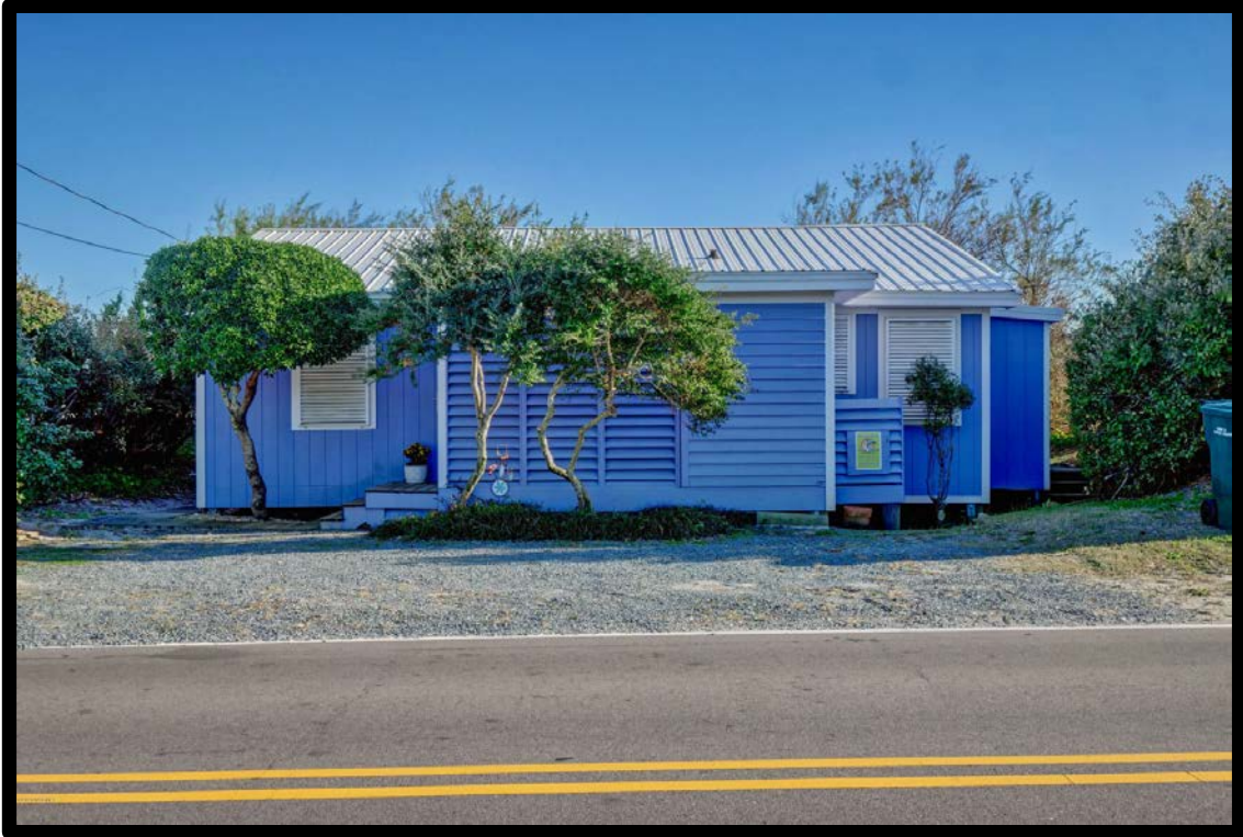
Front of porch from street – no view from inside
