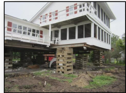
Elevation Raising Belhaven, NC
