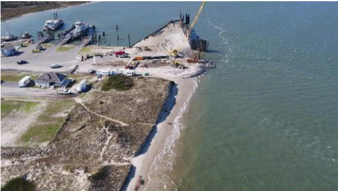
Photos of South Dock Erosion
