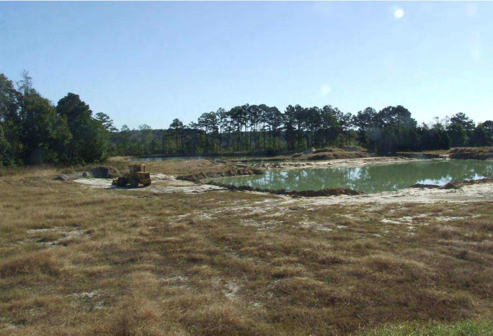
Authorized expansion of borrow pond TJ Land Development Property looking northeast Photograph taken on 20 October 2015
