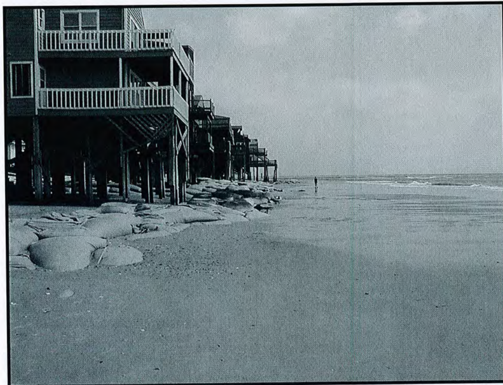
Figure 1. Sandbags at north end of North Topsail Beach (Sep 2005). (Note these sandbags no longer exist as they fronted buildings that were located seaward of the present structures north of Topsail Reef that were subsequently demolished.)
