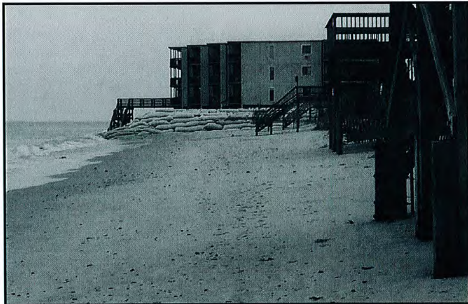
Photo 8. Sandbags revetment at Topsail Reefs Building 1 (Sep 2014).
