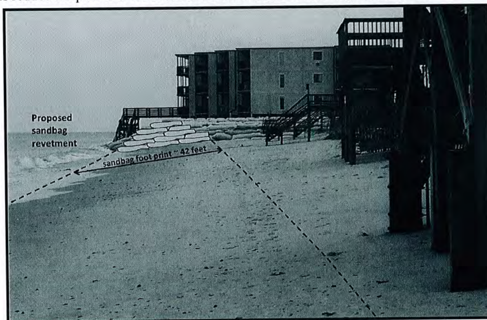
Figure 4. Schematic of tie-in of proposed sandbag revetment to the existing Topsail Reef sandbag revetment.
