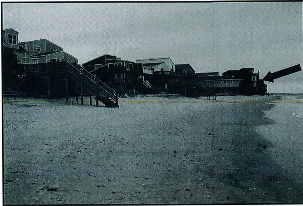
Photo No. 3a. Condition as of September 14, 2014.
