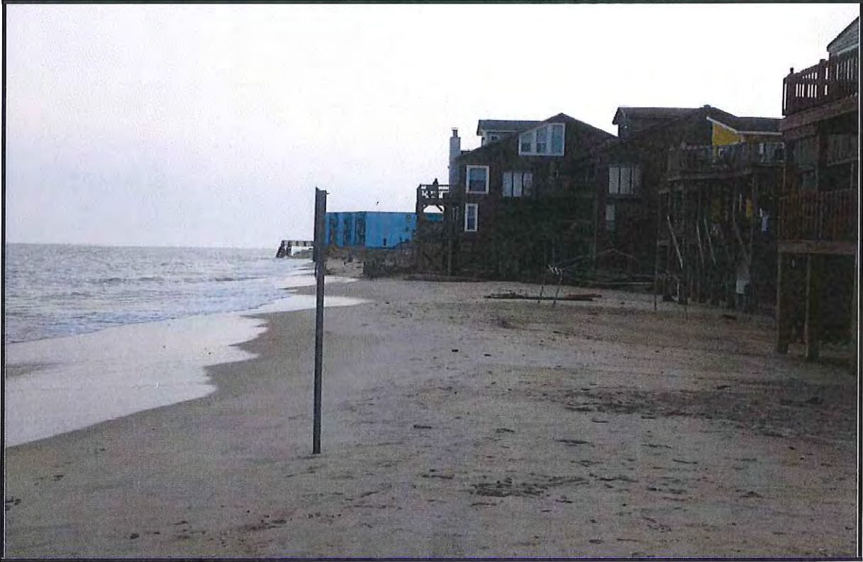
EXHIBIT 5: View looking south toward Topsail Reef Building #1 – August 7, 2014.
