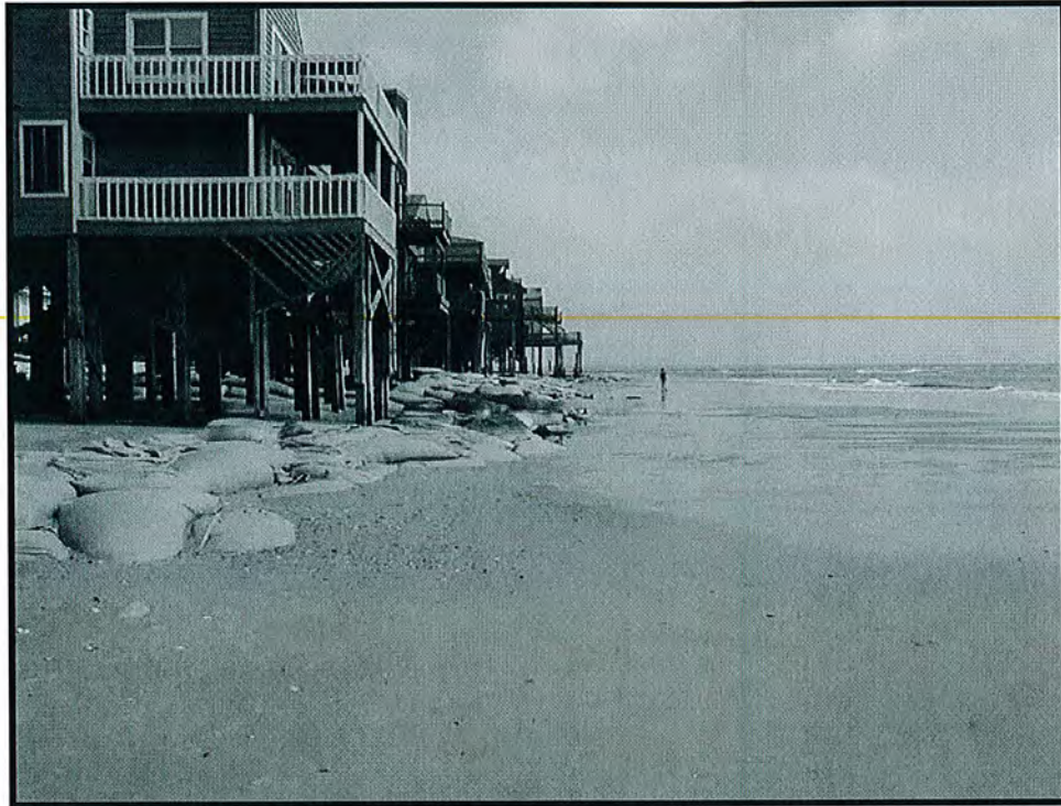
Photo 7. Example of failed sandbag revetment on north end of North Topsail Beach. Photo taken in September 2005. All of these sandbags and structures, which were located seaward of the present row of homes north of Topsail Reef, have been removed.
