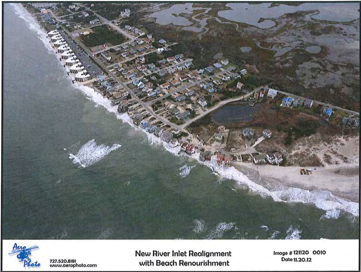
EXHIBIT 1: Pre-Nourishment – November 2012. The eight buildings in the upper left of the photo are the Topsail Reef Condominiums.
