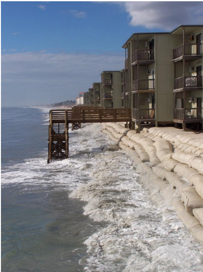
Before Phase 1 Construction
