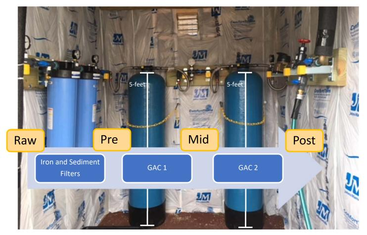
Sampling of pilot study GAC systems began in May 2018. Samples are collected at three sampling points: **raw**, **mid** which is after the first GAC filter, and **post** which is after the second GAC filter.
