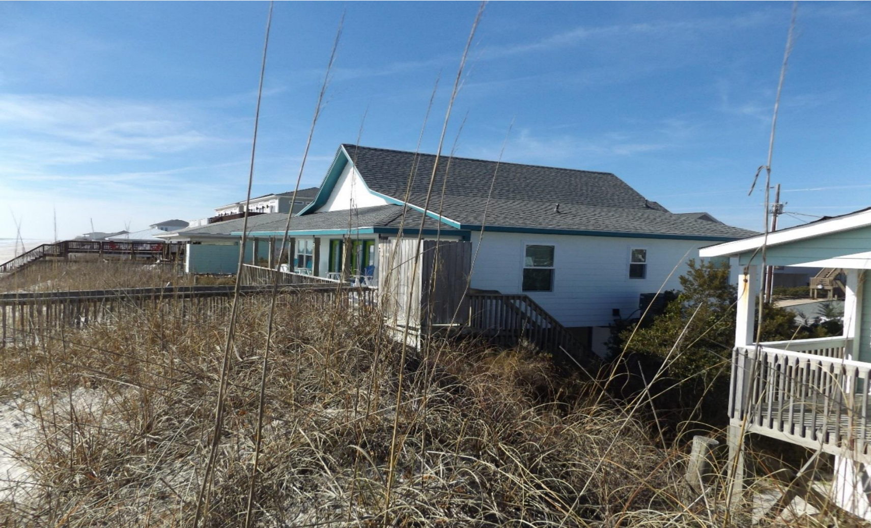
View of Petitioner's property looking South
