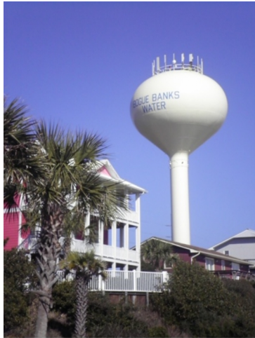
Bogue Banks Water Tower Image Source: HCP, Inc.
