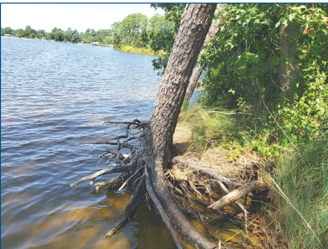
Southern Shoreline Erosion (looking west) August 8, 2019
