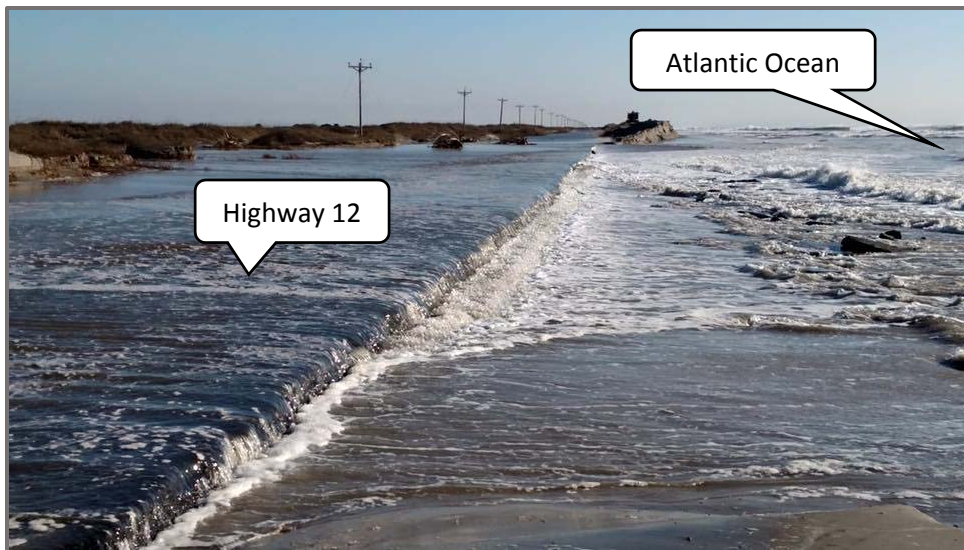
Figure 6. Dune breach and overwash along N.C. 12 following a February 7, 2016 storm. Photo: Hyde County Emergency Services
