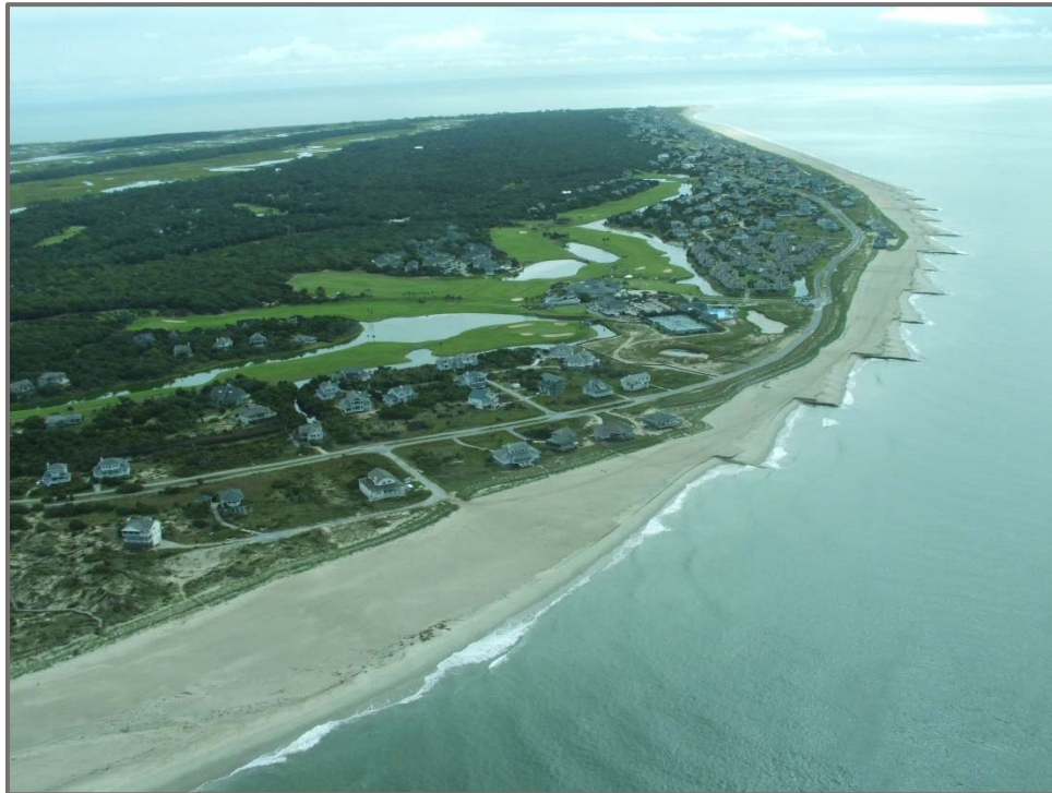
Figure 10. Groyne field installed in 2005 at Village of Bald Head Island. Photo: NCDCCM, 2007
