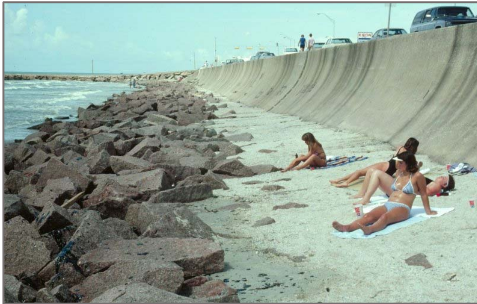
Figure 13. Seawall in Galveston, Texas. Photo: USACE, 2005
