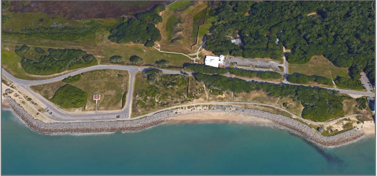
Figure 14. Fort Fisher State Park, N.C. rock revetment. Photo: NCDCM
