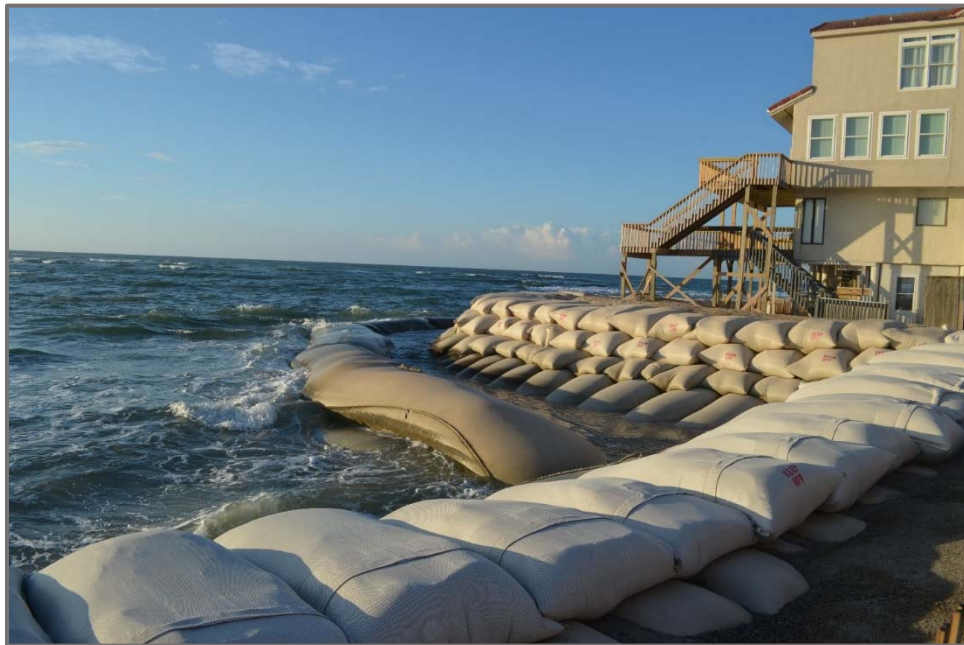
Figure 23. Sandbag structures at North Carolina's North Topsail Beach have been successful in providing short-term home protection from erosion at the expense of losing a sandy beach. Photo: NCDCEM, 2015
