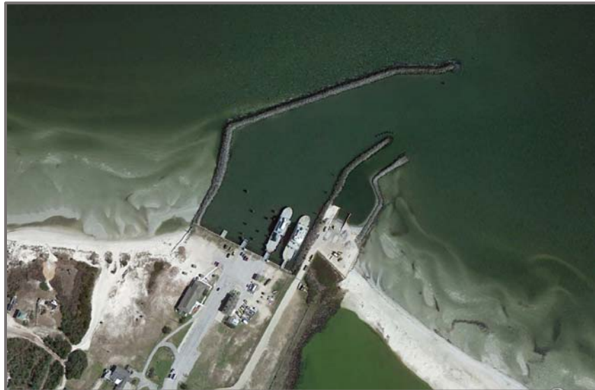
Figure 20. Breakwater connected to the beach at Cedar Island, N.C. ferry terminal. Photo: NCDWM, 2012
