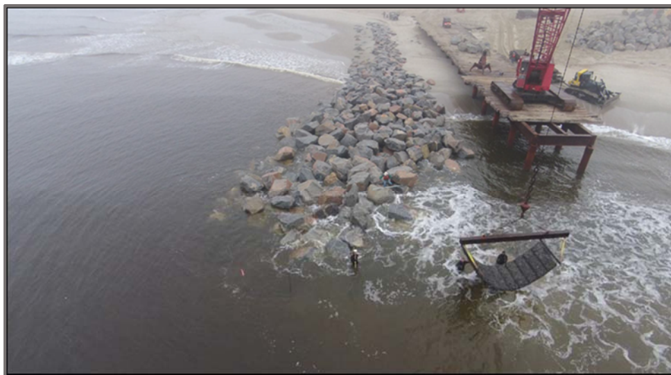
Figure 11. Terminal groin being installed at the Village of Bald Head Island in 2015. Photo: Village of Bald Head Island, 2015
