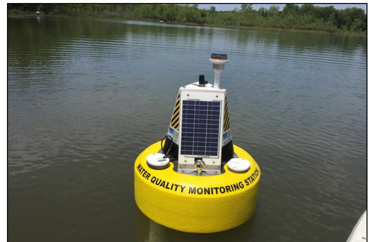
Automated Monitoring Equipment
