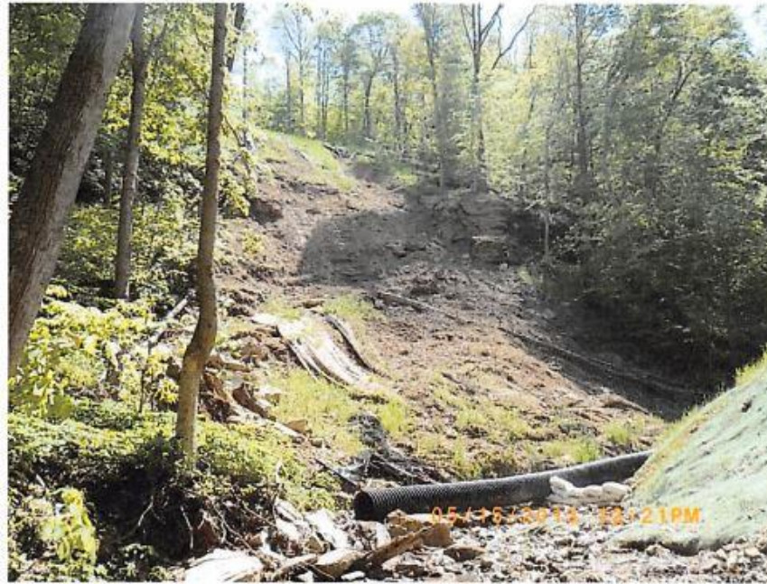
Photo 3: N 39° 52.3772' W 80° 41.1271' Bartletts Run. Flume pipe, sand bags and slip material in stream.
