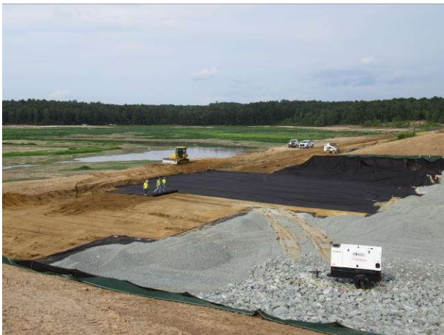
Upstream area of breach covered by fabric
