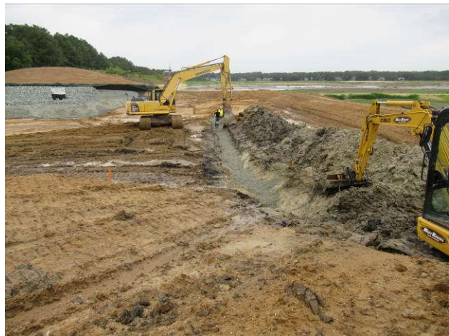
Dewatering trench filled with bedding stone
