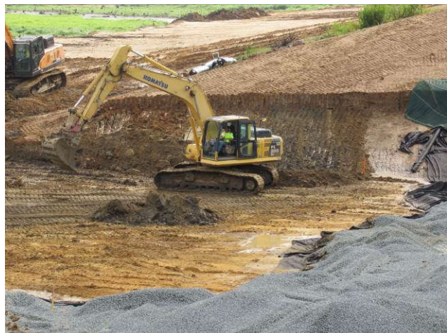
The transition wall is extended upstream
