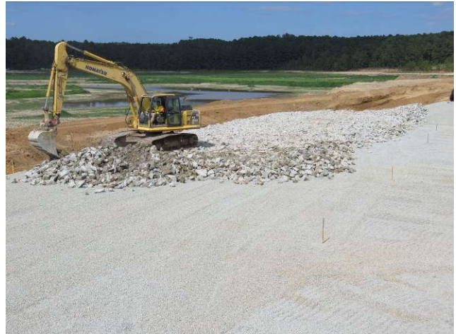
Riprap is placed along the upstream end of the breach
