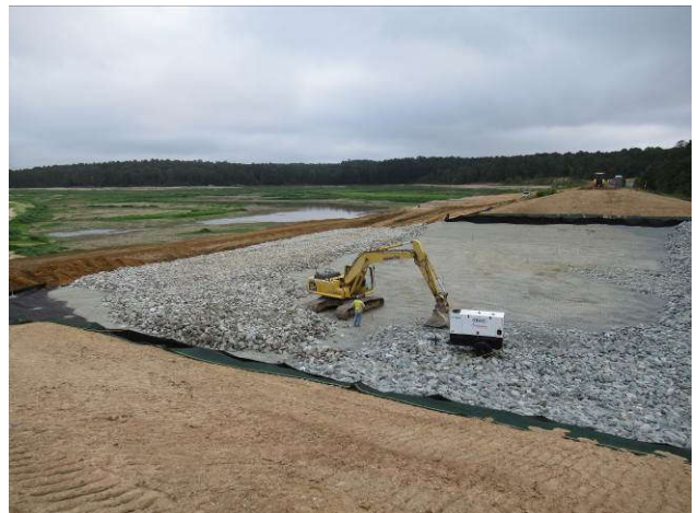
Riprap is tied to the existing riprap downstream
