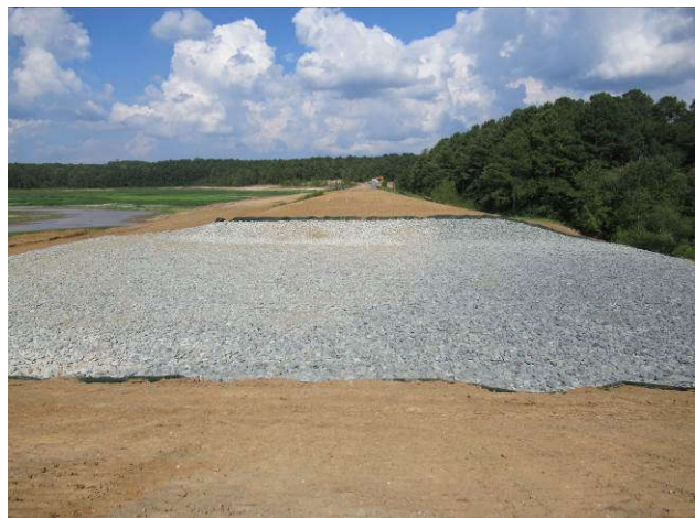
The transition wall is extended upstream
