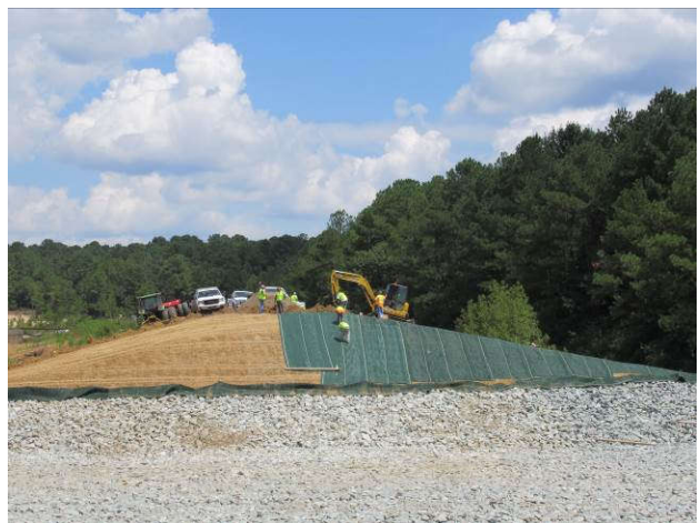
Turf mat installation partially complete on the left slope
