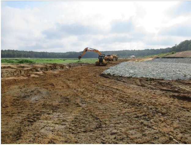
Cofferdam being removed down to the elevation of the breach
