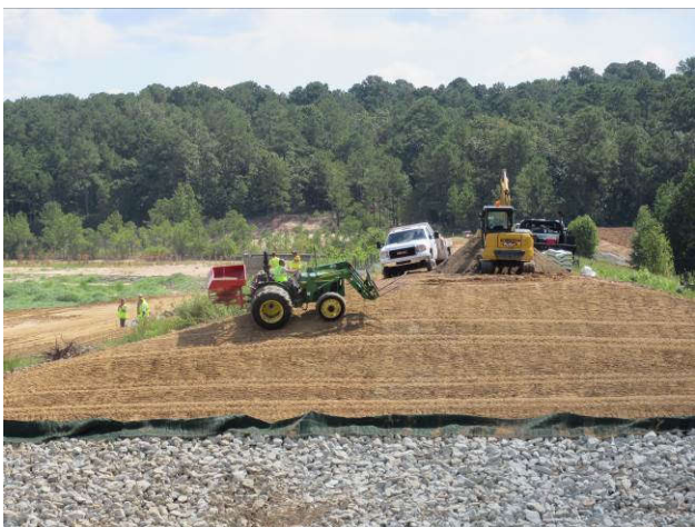
Seeding begins on the left slope
