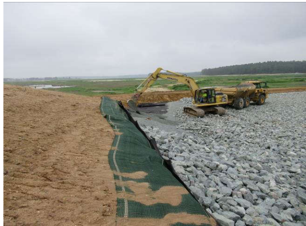
Upstream right corner covered with riprap
