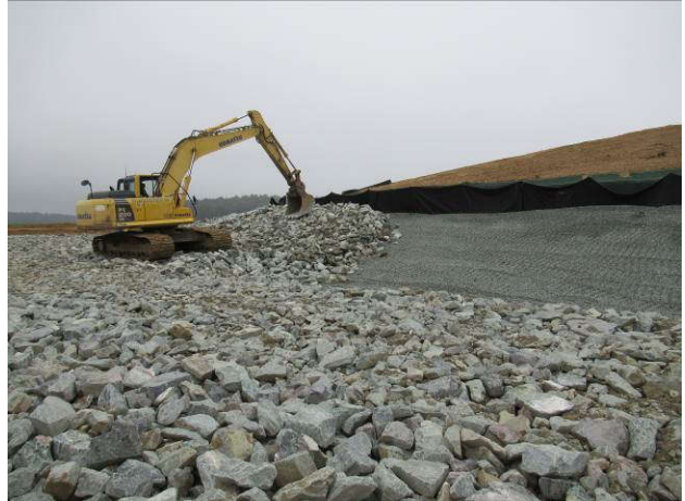
View of left slope being covered by riprap
