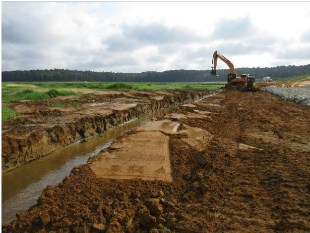
View of the restored channel upstream of the breach
