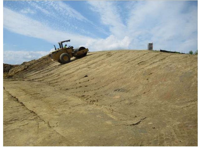
Compaction of the slope onto the abutment
