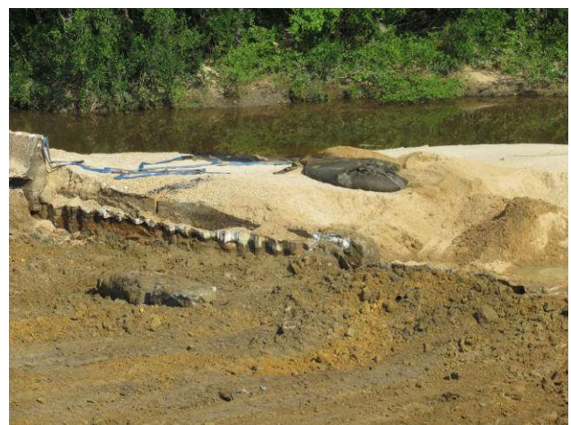
Cut and fill to the sheetpile walls
