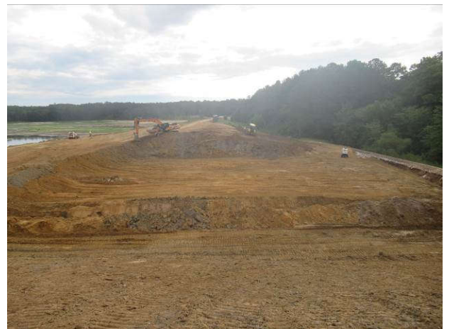
View of spillway at beginning of the week
