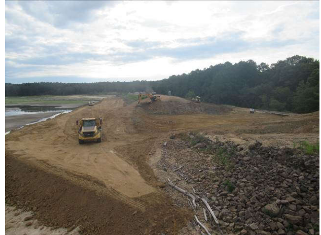
View of cofferdam at beginning of the week
