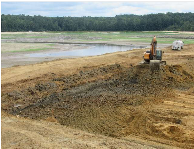
The upstream spillway being cut to grade
