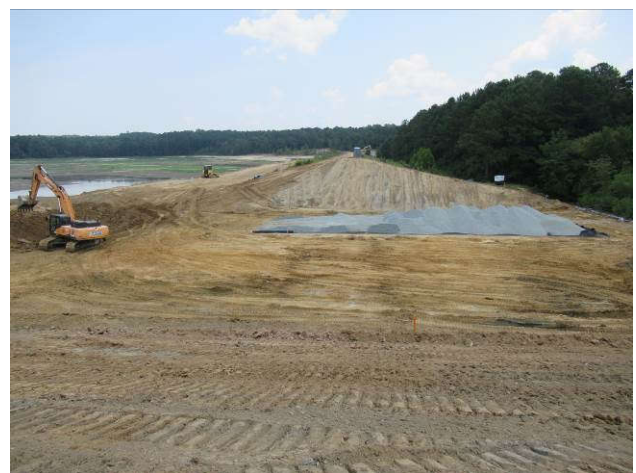
View of the spillway at end of the week
