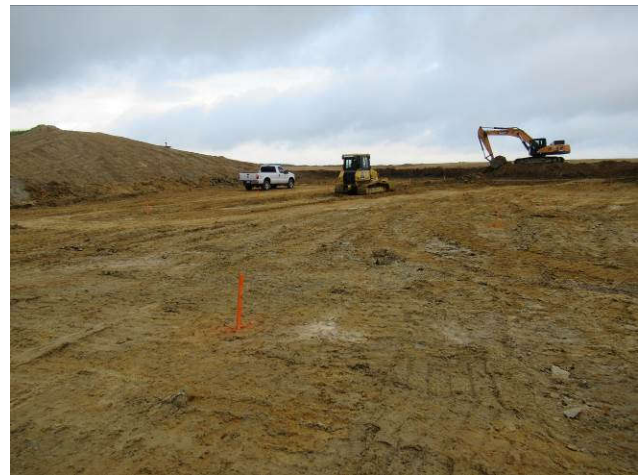
Preparing a section for final grade
