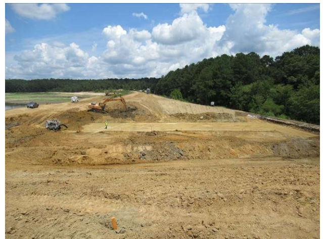
Section compacted and inspected
