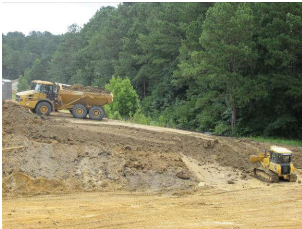
The slope onto the abutment being filled to grade
