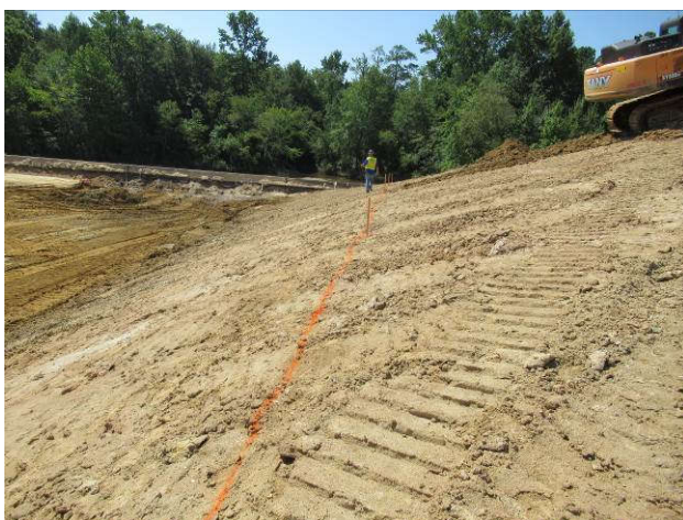
Surveying slope for cut and fill to grade
