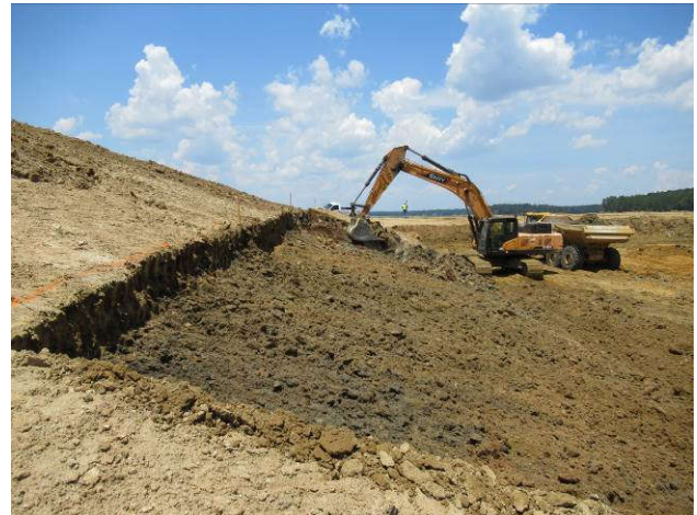
View of the slope being cut by the excavator
