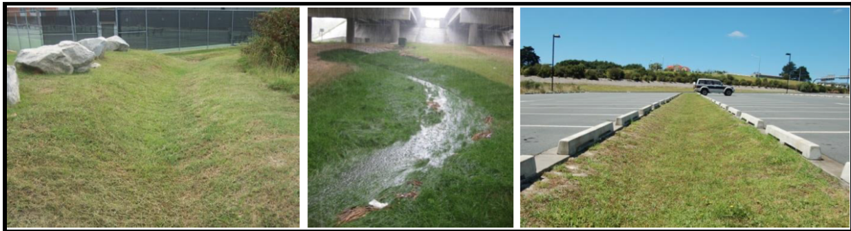
Figure 1: Swales are used world-wide, such as those (left to right) on NCSU campus (Raleigh, NC), under a bridge deck in Knightdale, NC, and serving a parking lot in Albany, New Zealand. 1
