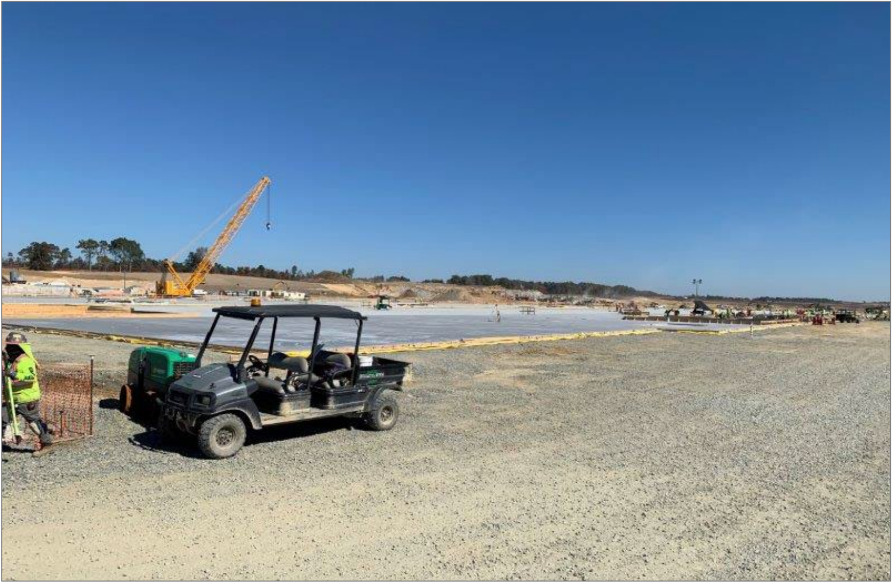
Toyota Battery Manufacturing North Carolina site - October 24, 2022
