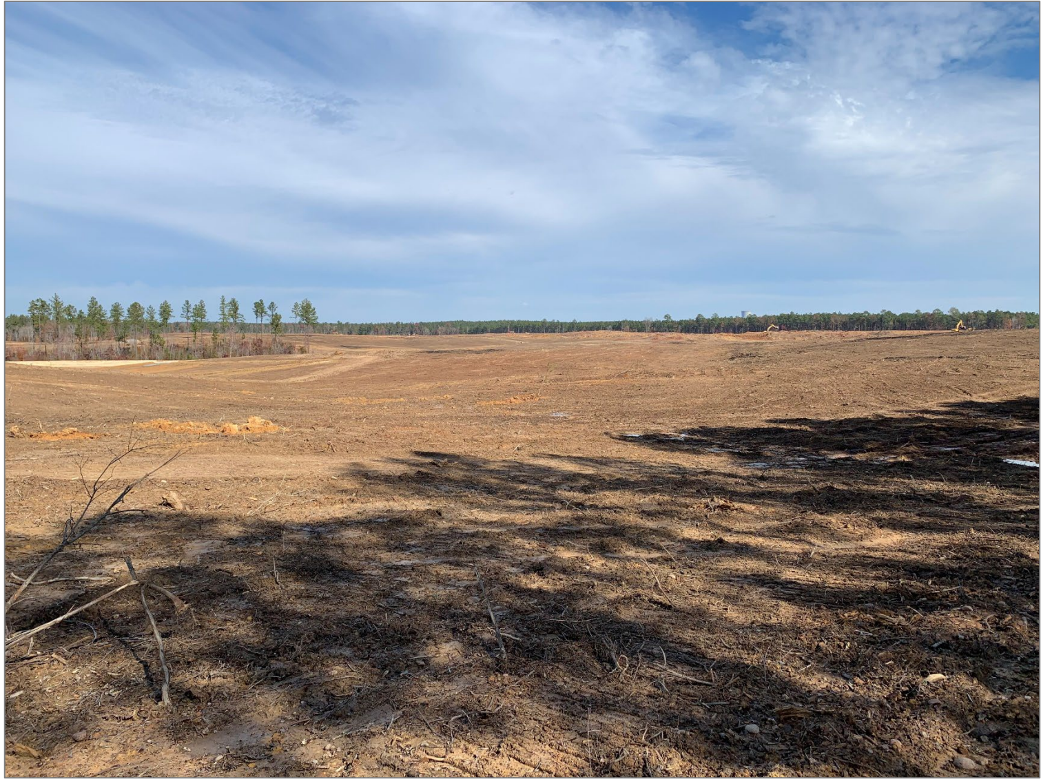
Site of VinFast EV Plant, Triangle Innovation Point – November 2, 2022
