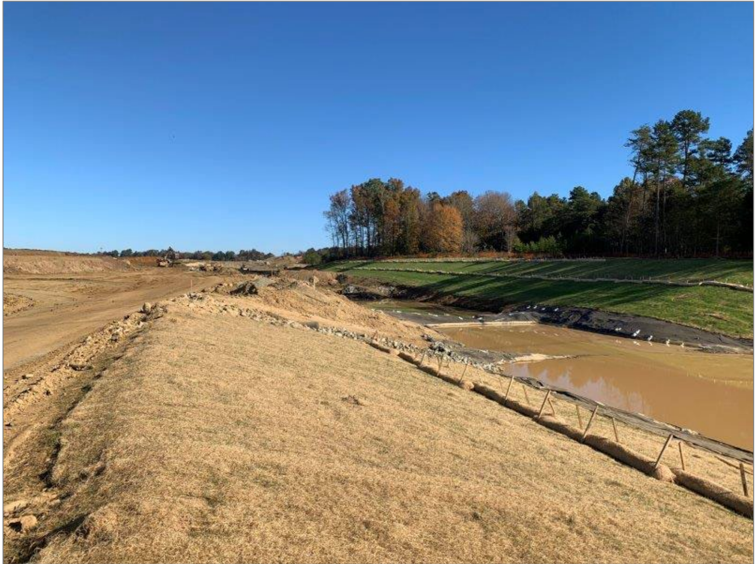
Toyota Battery Manufacturing North Carolina site - October 24, 2022
