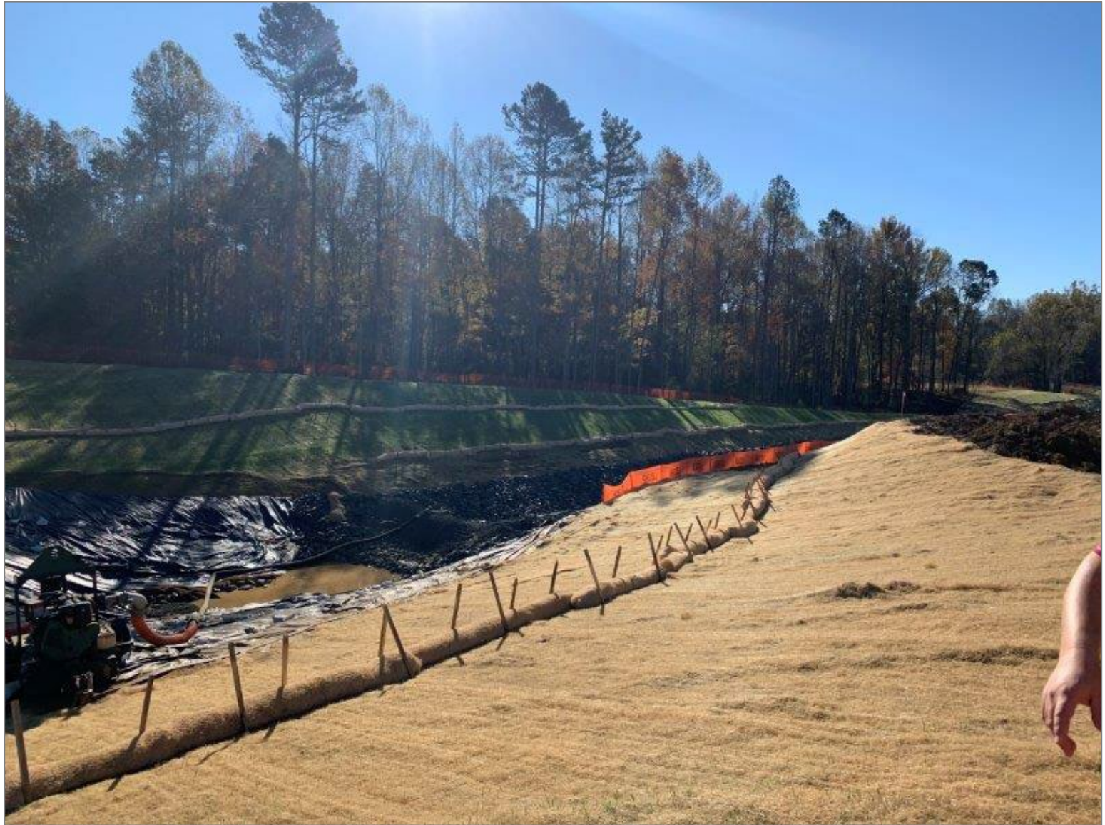
Toyota Battery Manufacturing North Carolina site - October 24, 2022
