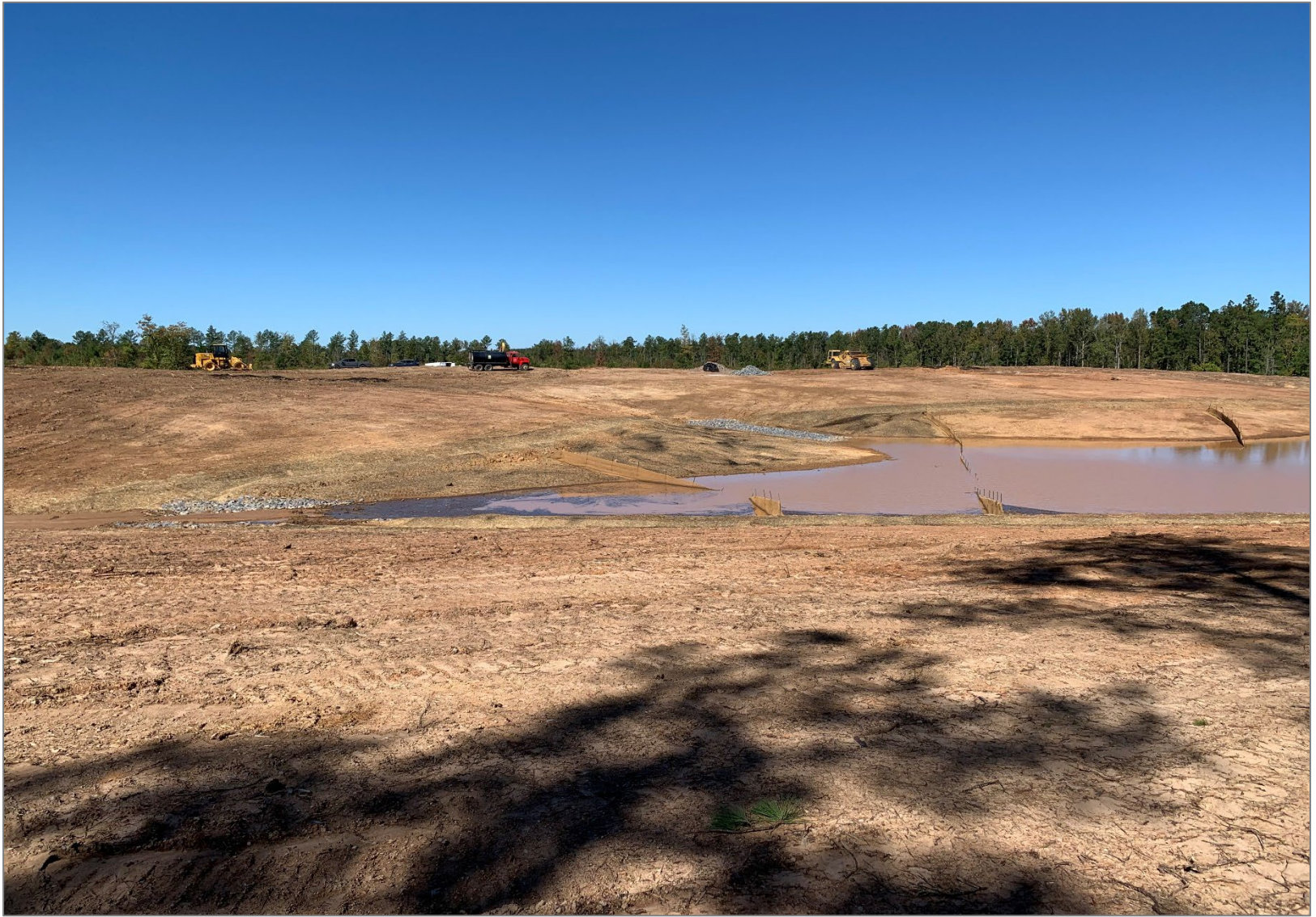
Site of VinFast EV Plant, Triangle Innovation Point – November 2, 2022
