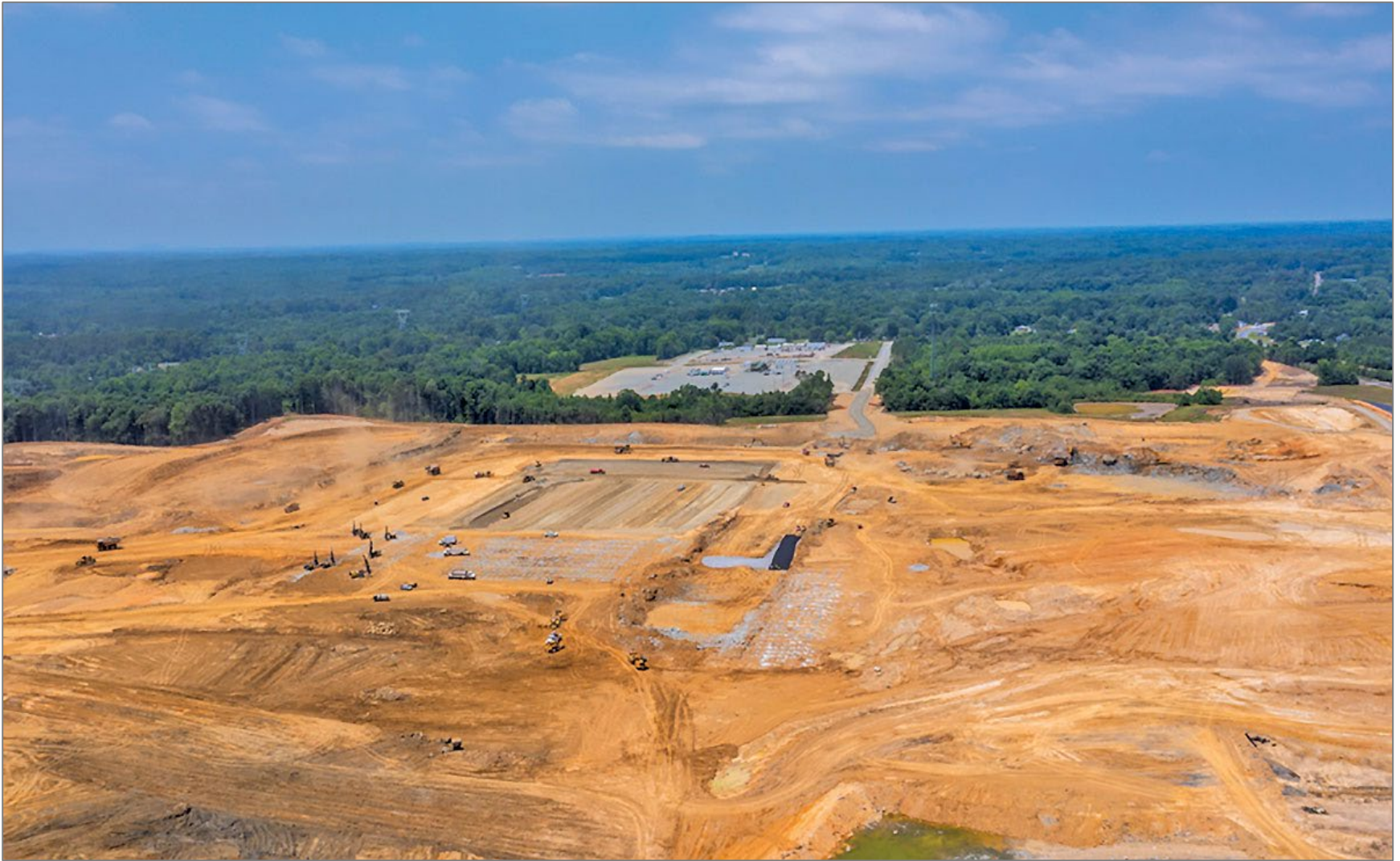
Toyota Battery Manufacturing North Carolina site - June 2022
