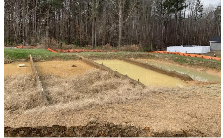
Baffles 1,2 and 3- This basin is a good example of the baffles functioning as water cleared as it moved toward the skimmer. Photo Credit NCDEQ Staff
