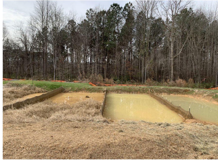
Baffles 1,2 and 3- This basin is a good example of the baffles functioning as water cleared as it moved toward the skimmer. Photo Credit NCDEQ Staff
