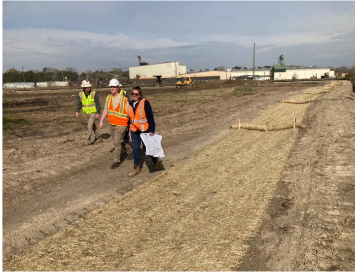
Wattles around perimeter of site - Photo Credit NCDEQ Staff
