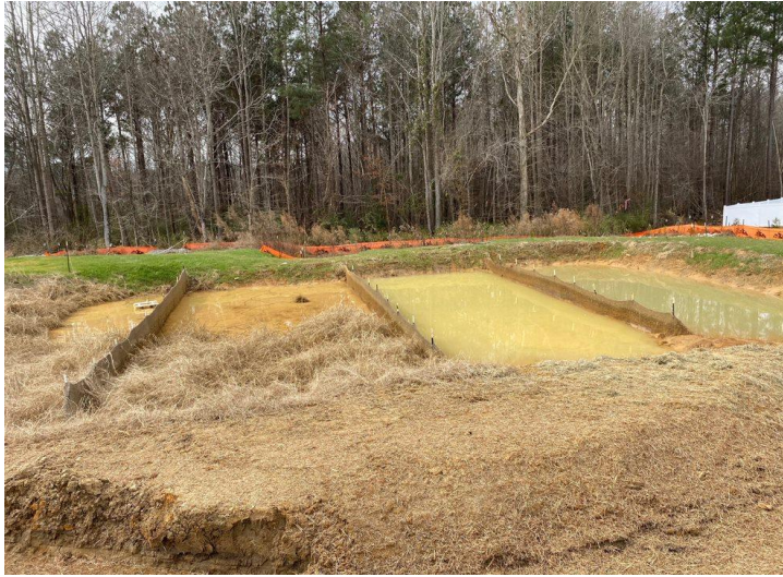
Baffles 1,2 and 3- This basin is a good example of the baffles functioning as water cleared as it moved toward the skimmer. Photo Credit NCDEQ Staff
