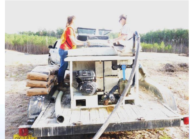
Sprayed Concrete (PosiShell)
