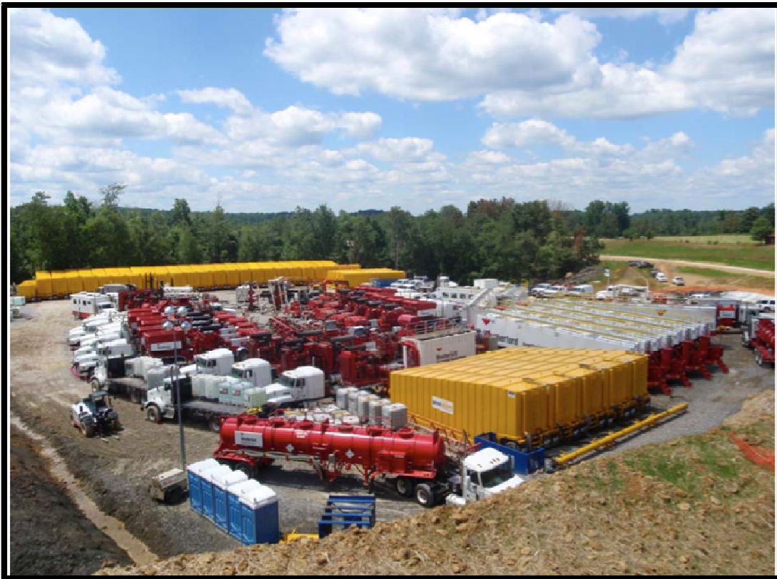
Figure 6-9. Hydraulic Fracturing in Upshur Valley, West Virginia (Marcellus region)
