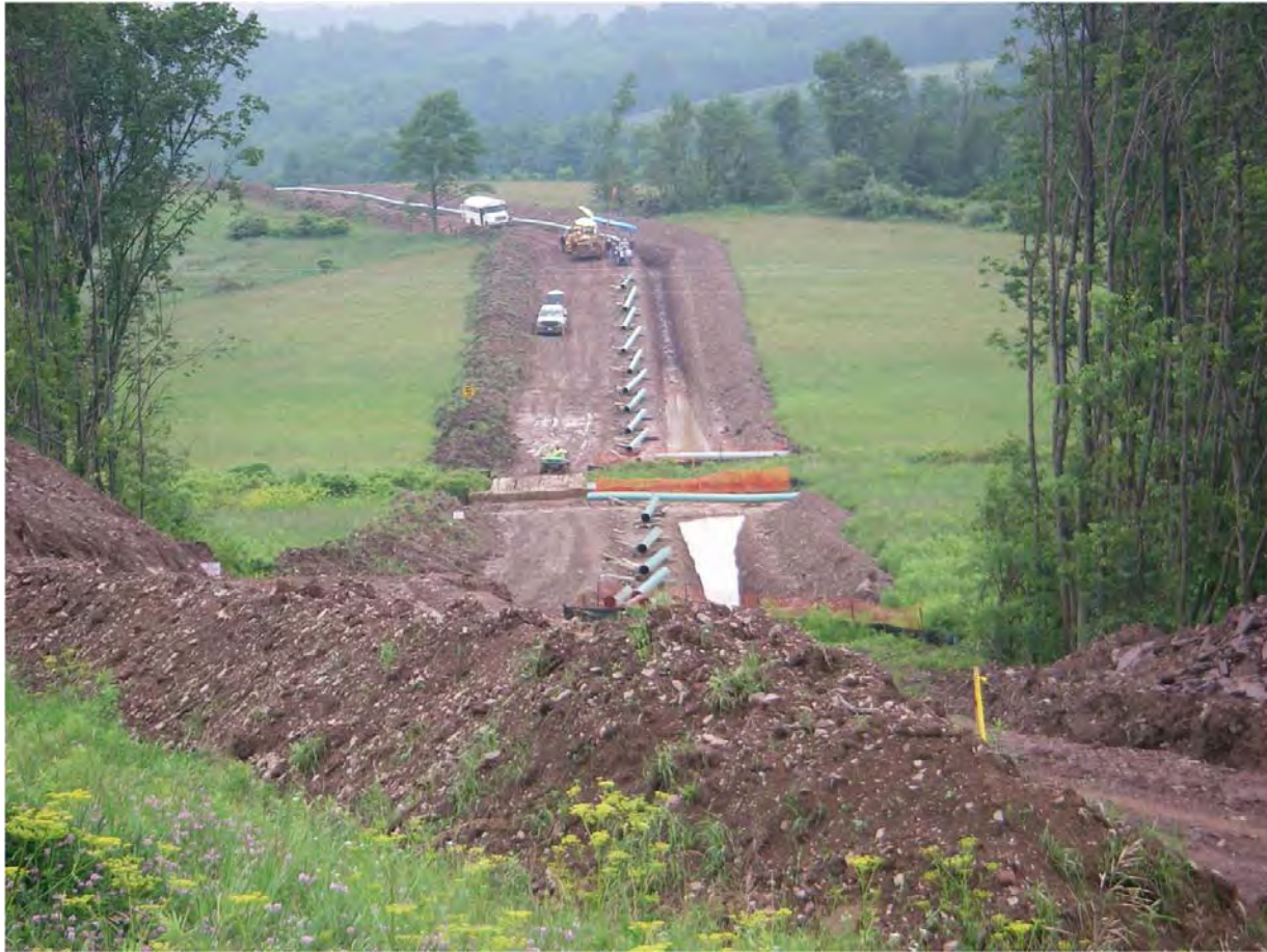
Figure 3-12. Construction of Underground Pipeline
