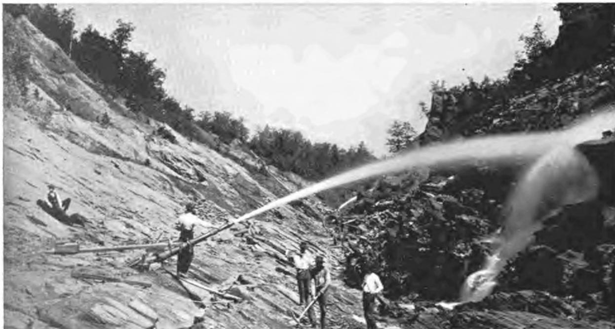
DAHLONEGA METHOD OF MINING, SHOWING GIANT AND GROUND SLUICE.
