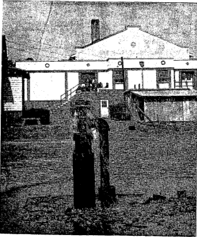
A.—Flowing well at Bullocks School in Wilson County. This well is drilled in granite and is 159 feet deep. When drilled, the flow was 60 gallons a minute, and the water would rise 12 feet above the surface.
