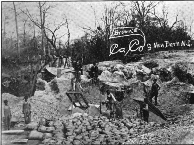
A. Working Marl deposits with hand labor
