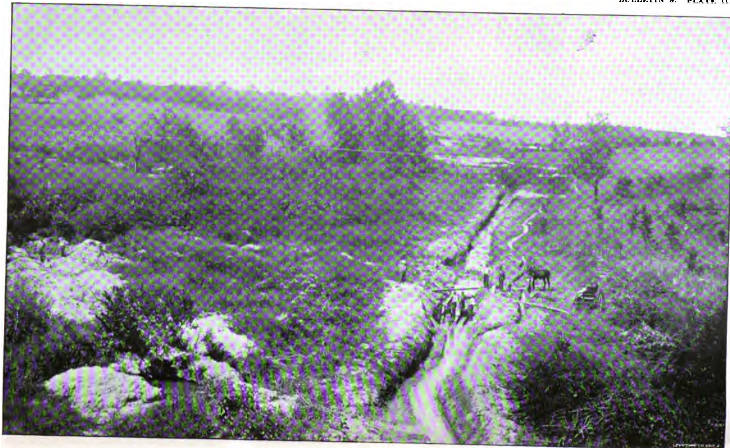
WASHING GRAVEL AND SAND IN STREAM BEDS FOR MONAZITE, LATTIMORE MINE.
