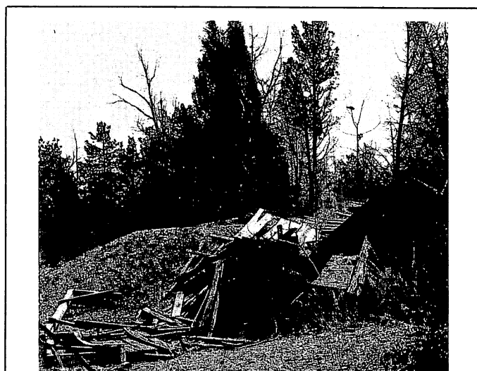
Plate 9A. Collapsed headframe over Barnhardt Shaft
