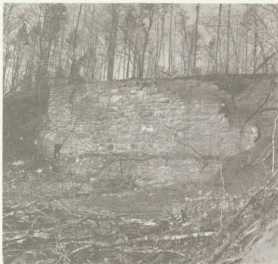
Plate 5B. Remains of furnace at the Buckhorn Mine
