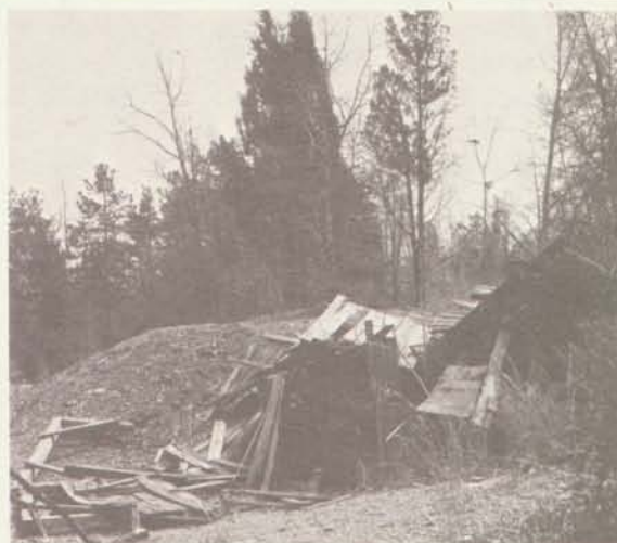
Plate 9A. Collapsed headframe over Barnhardt Shaft
