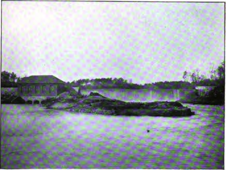
A DAM AND POWER-HOUSE, SALUDA RIVER, PELZER, S. C.
