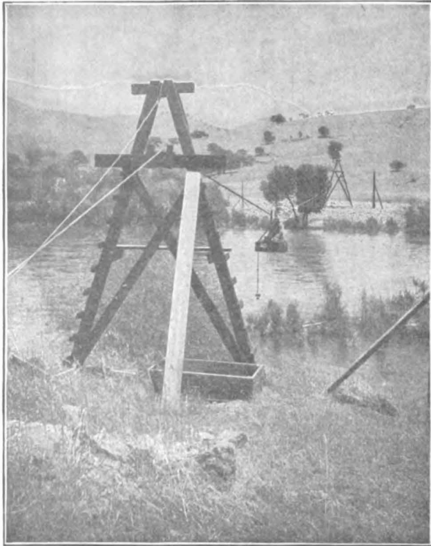
FIG. 1a. A TYPICAL CABLE STATION.
