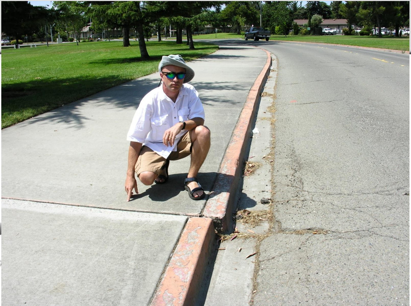
Strike Slip Fault – Hayward Fault, Fremont Ca
