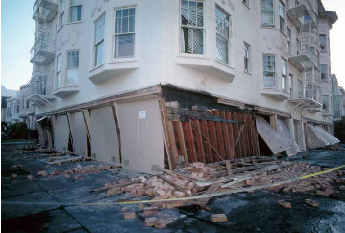
Figure 5. “Soft” or weak first story failure of a four-story building in San Francisco damaged by the October, 1989 Loma Prieta earthquake. In this case the weak story is caused by reduced shear wall strength and lack of diagonal bracing related to constructing parking garages (note garage doors) in the first story of the building.
