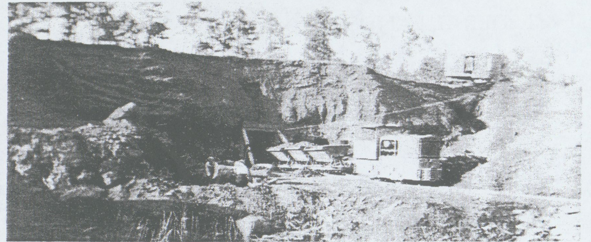
Removing overburden at the Portis Mine, Franklin Co., 1935. (NCGS Bulletin 38.)
