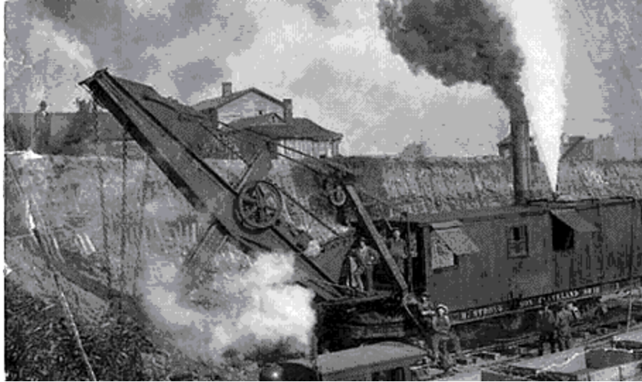
Figure 6 “Steam Shovel in use in one of Berea’s quarries.” Published by D.A. Beswick, Berea, Ohio. Dorothy M. McKelvey Collection, Berea Historical Society. Used with permission of the Berea Historical Society.
