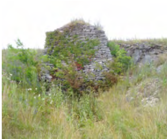
FIGURE 3c A brick, silo-type, lime kiln.
