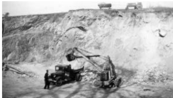
FIGURE 12 View of Kipps quarry with three-quarter swing Fortson shovel loading 1934 Ford dump-truck. Above quarry face a 1942 Oliver tractor powers an air compressor used to drill holes for bench shots.
