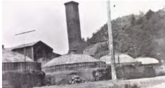
FIGURE 2c Old image of Marion Brick Company beehive kilns, along Staley Creek in Smyth County, VA (Byrd and Williams, 2005).
