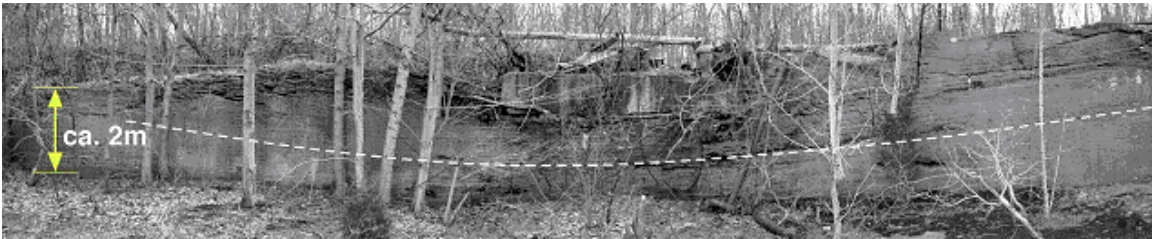
FIGURE 2 (Top) Wall of the Cleveland Quarries Company's Quarry No. 6, ca. 1950. Note the channel near the top of the wall. This and similar features (delineated by dashed line in bottom illustration from south wall of a quarry just to the south) were probably associated with the westward migration of fluvial environments over coastal and nearshore sediments as sea level fell. Photograph courtesy of Cleveland Quarries.
