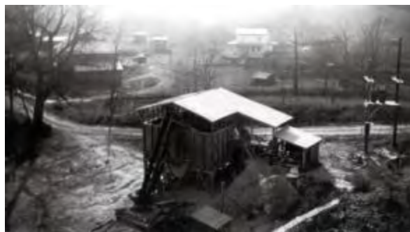
FIGURE 13 Kipps' mill with new REA electrical power substation at right edge of photograph.
