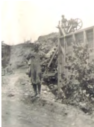
FIGURE 8 First storage bin (50-ton capacity) after completion, with Elmer A. Kipps in foreground and 11-year-old Elmer C. Kipps with shovel of milled lime from the J.B. Hammer Mill.
