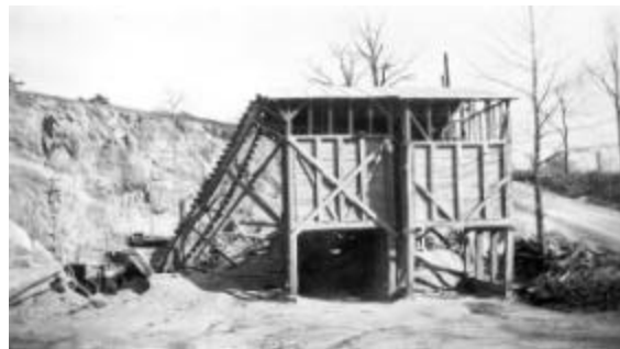
FIGURE 10 View of twin storage bins with elevator feed to cylinder screen housed above 1st bin (100-ton capacity) and Stover Hammer Mill above second bin (50-ton capacity). The hammer mill was powered a by diesel Titan tractor, located behind bins.
