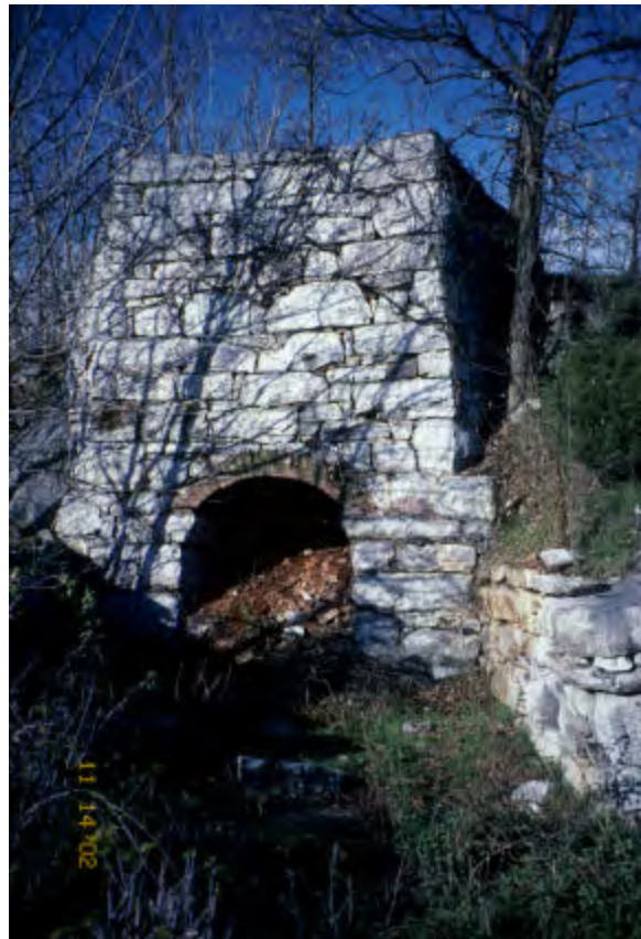
FIGURE 2 Meyers lime kiln, built in the early 1900s in Rockingham County, Virginia.
