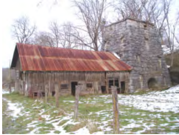
FIGURE 2b The Irondale Furnace was active from 1881-1893, along Francis Mill Creek in Wythe County, VA.
