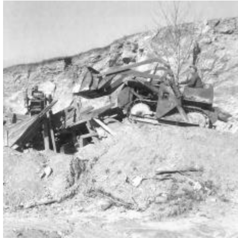
FIGURE 14 E.C. Kipps dumping International TD9 front-end loader into jaw-crusher in December 1959.
