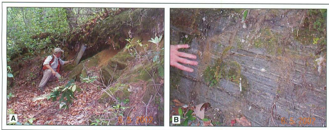
Figure 16. Bedrock exposed in the main scarp of the Toxaway River slide. A. Partly decomposed Toxaway Gneiss exposed in the main scarp of the Toxaway River slide. The down-dropped part of the slide is in the left foreground. B. Completely decomposed, mylonitic Toxaway Gneiss exposed in the main scarp of the Toxaway River slide. White, elongate porphyroclasts of potassium feldspar are flattened in the plane of the mylonitic foliation, delineated here by alternating light and dark banding. Photographs courtesy of Malcolm Schaeffer.
