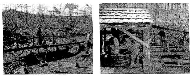
Figure 20. Log rockers and Chilean drag mill and rockers near Gold Hill, about 1896 (From Nitze and Wilkens, 1897).
