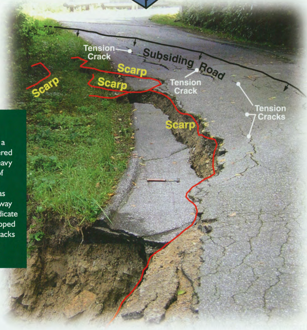
Figure 4 Main parts of a general landslide.
