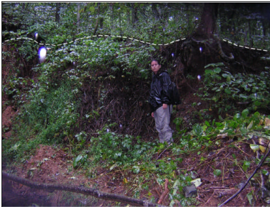
Figure 6. Top of older scarp (white dashed line) exposed at Site 1. Geologist is standing on down-dropped surface. This partially vegetated older scarp predates the new scarp formed by the August 22, 2005 slope failure (just southeast of this location shown in figure 5). The older scarp may have developed in the reported 1977 landslide deposits.
