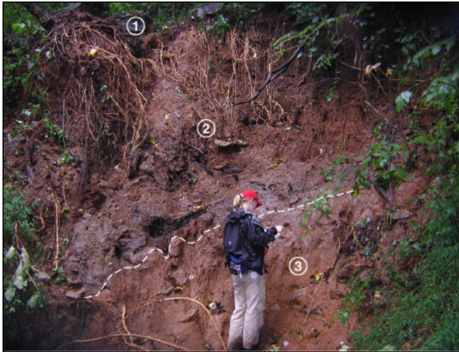
Figure 5. Head scarp of slope failure at Site 1. Deposit 1 – Rock boulders from airport construction on ground surface. Deposit 2 – Sand-silt-clay mixture with large fragments of organic debris. Deposit 3 – Colluvial hillslope deposit consisting of sandy, silty clay with gravel and cobbles. Portions of layers 1 and 2 may have been transported during the reported 1977 landslide.
