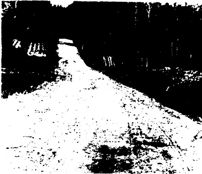
Portion of completed access road leading to Hamme Tungsten property
