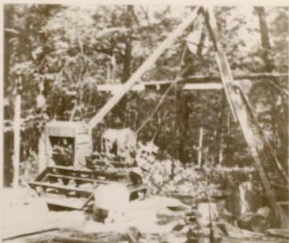
Setting up Sprague and Henwood Diamond Drill on Morton Property.
