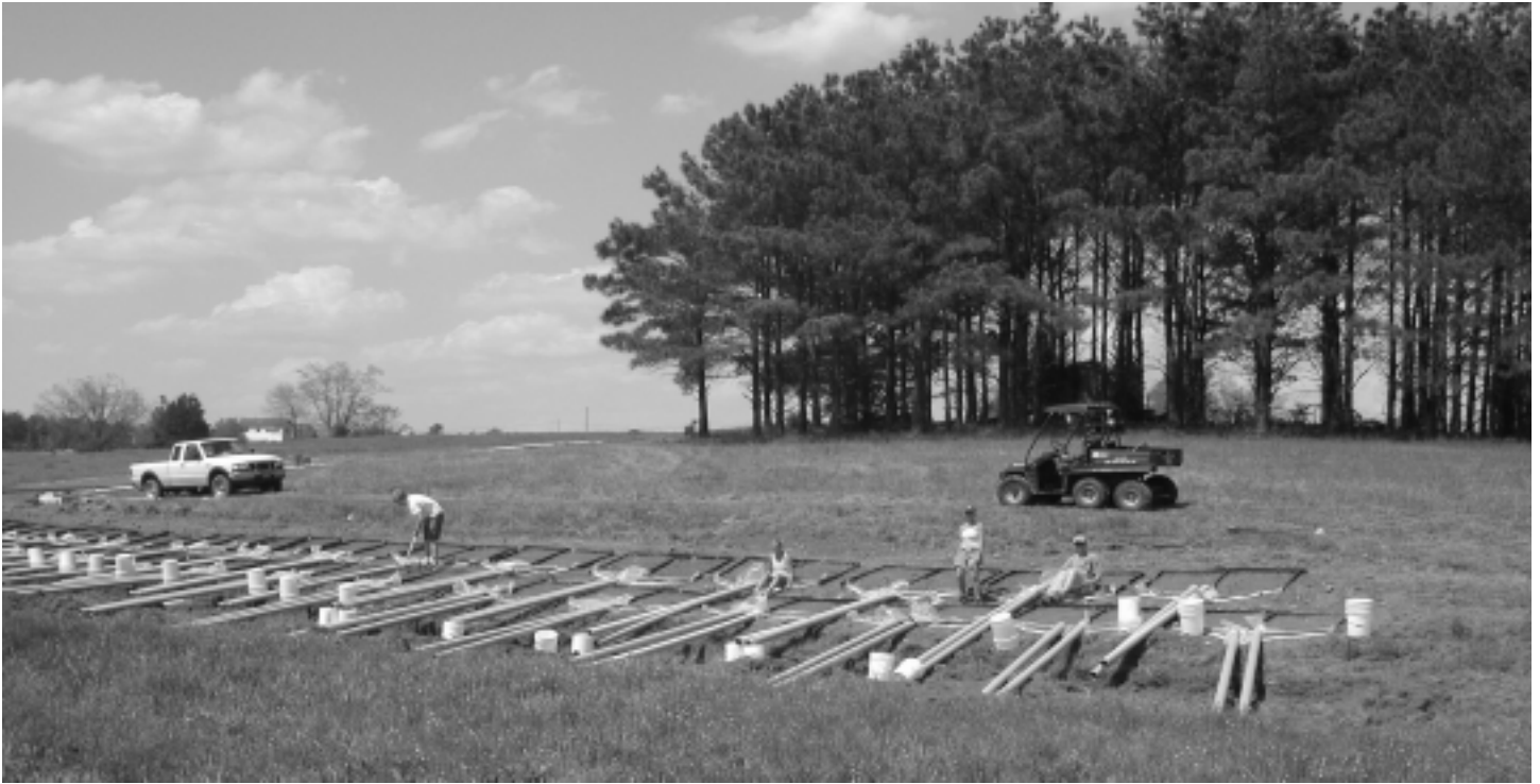
At the NCSU Sediment and Erosion Control Research Facility, Dr. Rich McLaughlin designed a research project to determine if PAMs can increase the effectiveness of ground covers and aid in grass establishment. Thirty-two plots were monitored for runoff, turbidity and biomass.
