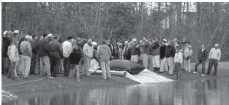
Demonstration of dirt bag filtering sediments out of stormwater pond using polymer injection system.
