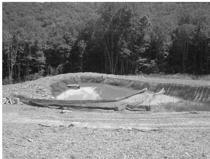
Practice Range Basin 1 in June 2004. Note the deposition of sediment behind the baffles, particularly the second baffle after the first one was overtopped.
